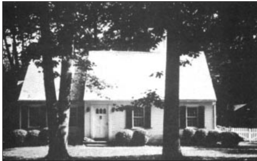
Figure 2-1 This house near Atlanta was flooded several times. During the largest flood, the water reached as high as 2 feet above the first floor.
