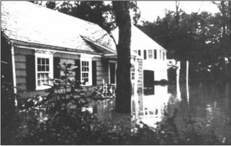
Figure 2-3 Now the house (in the background) is protected from flooding, unlike the flooded house in the foreground.
