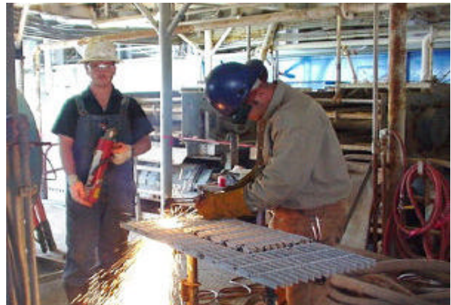
Fig. 1. Hot work - welding
