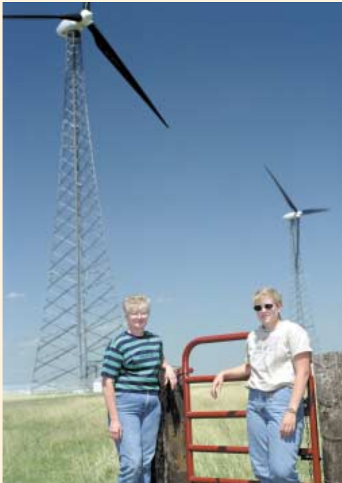
The twin turbines near Springview, Nebraska, generate enough electricity annually to serve 700 to 800 residential customers.
