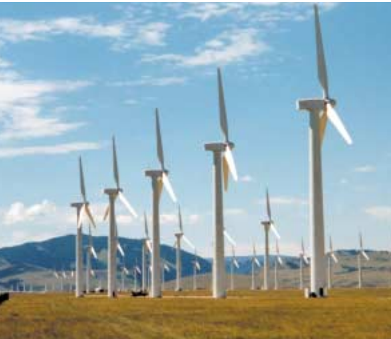
Sixty-nine turbines at Foote Creek Rim near Arlington, Wyoming, have 41 MW of generating capacity.
