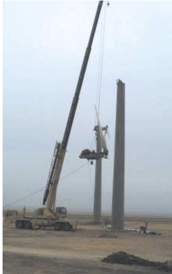
Researchers from Sandia National Laboratories instrument three 52-foot-diameter turbines mounted on 72-foot towers to gather load and wind inflow information.
