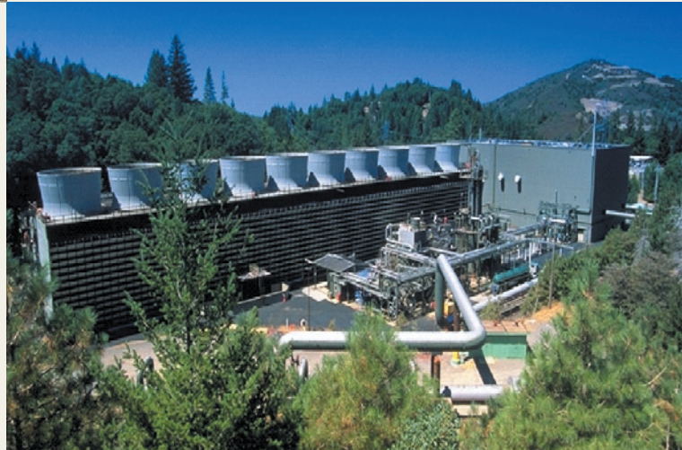
Pacific Gas and Electric Company (PG&E)
