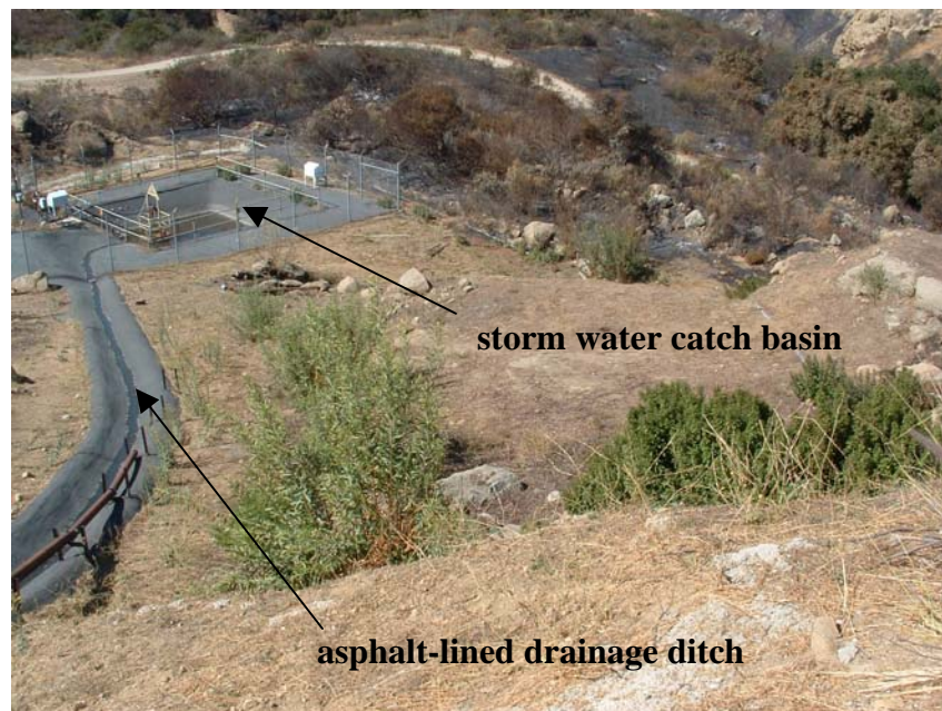
Figure 4.3 – Asphalt-Lined Drainage Ditch in Survey Unit 8 (Looking West)
