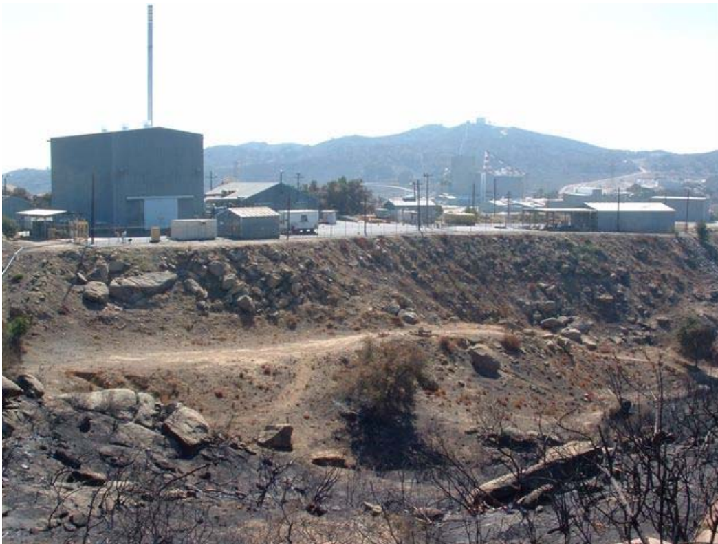
Figure 1.2 – Area of Interest on North Side of RMHF Perimeter (Looking South)
