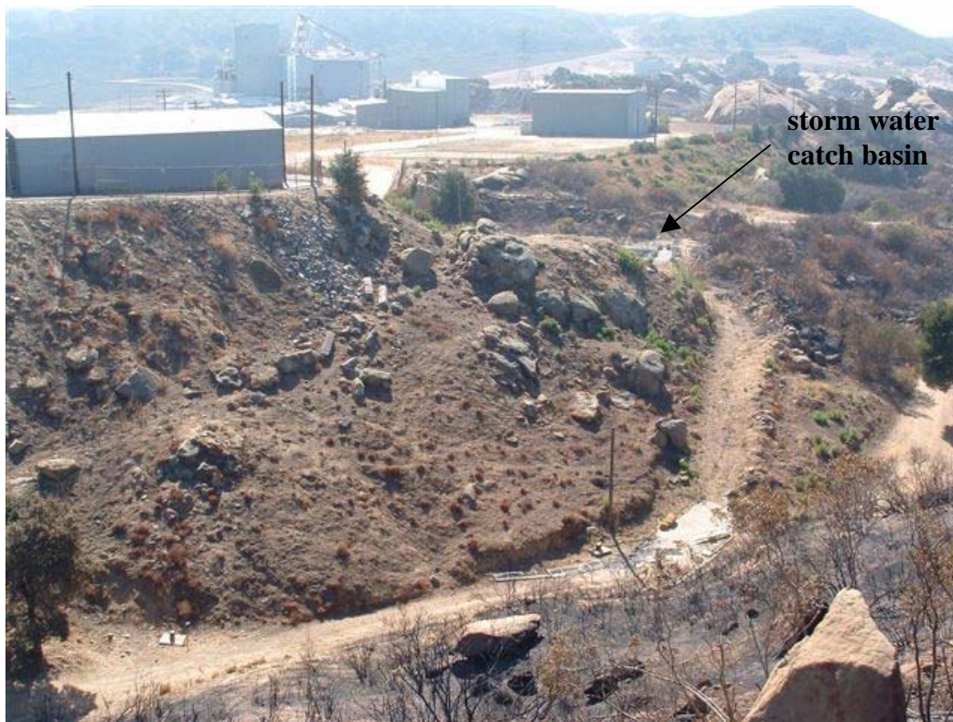
Figure 1.3 – Area of Interest on West Side of RMHF Perimeter (Looking Southwest)
