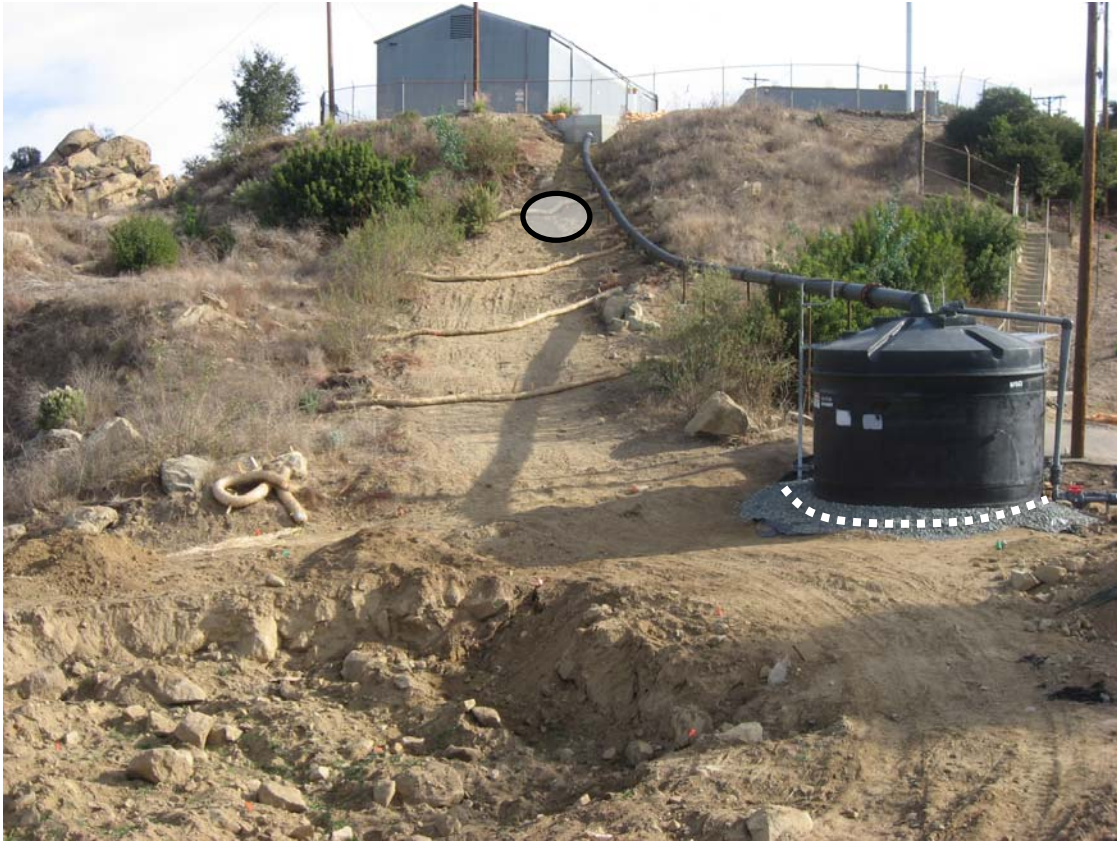
Figure 1.2 Site 4614 (View of Drainage Channel)
