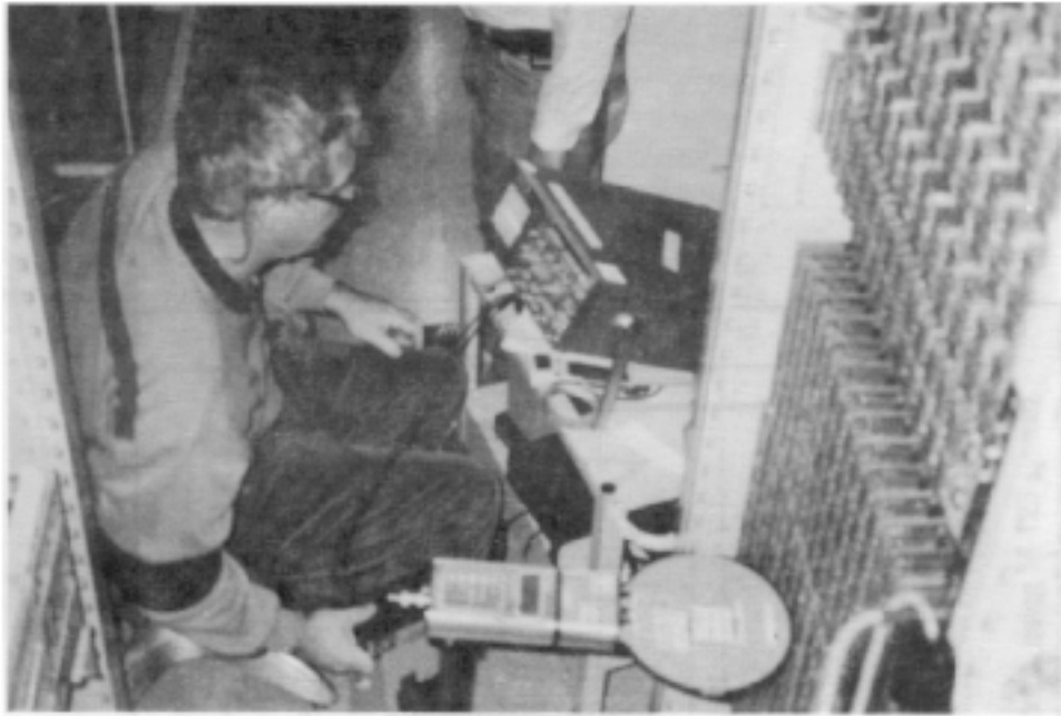
FIGURE 9. Illustration of "capturing" magnetic field transients from switching equipment.
