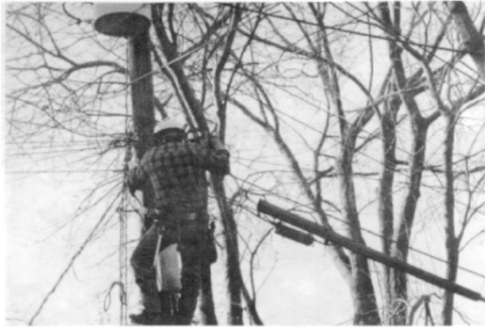
FIGURE 14. NYNEX worker on pole with a gasoline powered drill. Drill time was approximately 2 minutes. EMDEX meter was positioned around neck.
