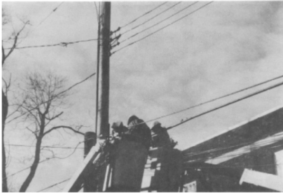
FIGURE 19. Splicers in boom installing new cable on shared pole
