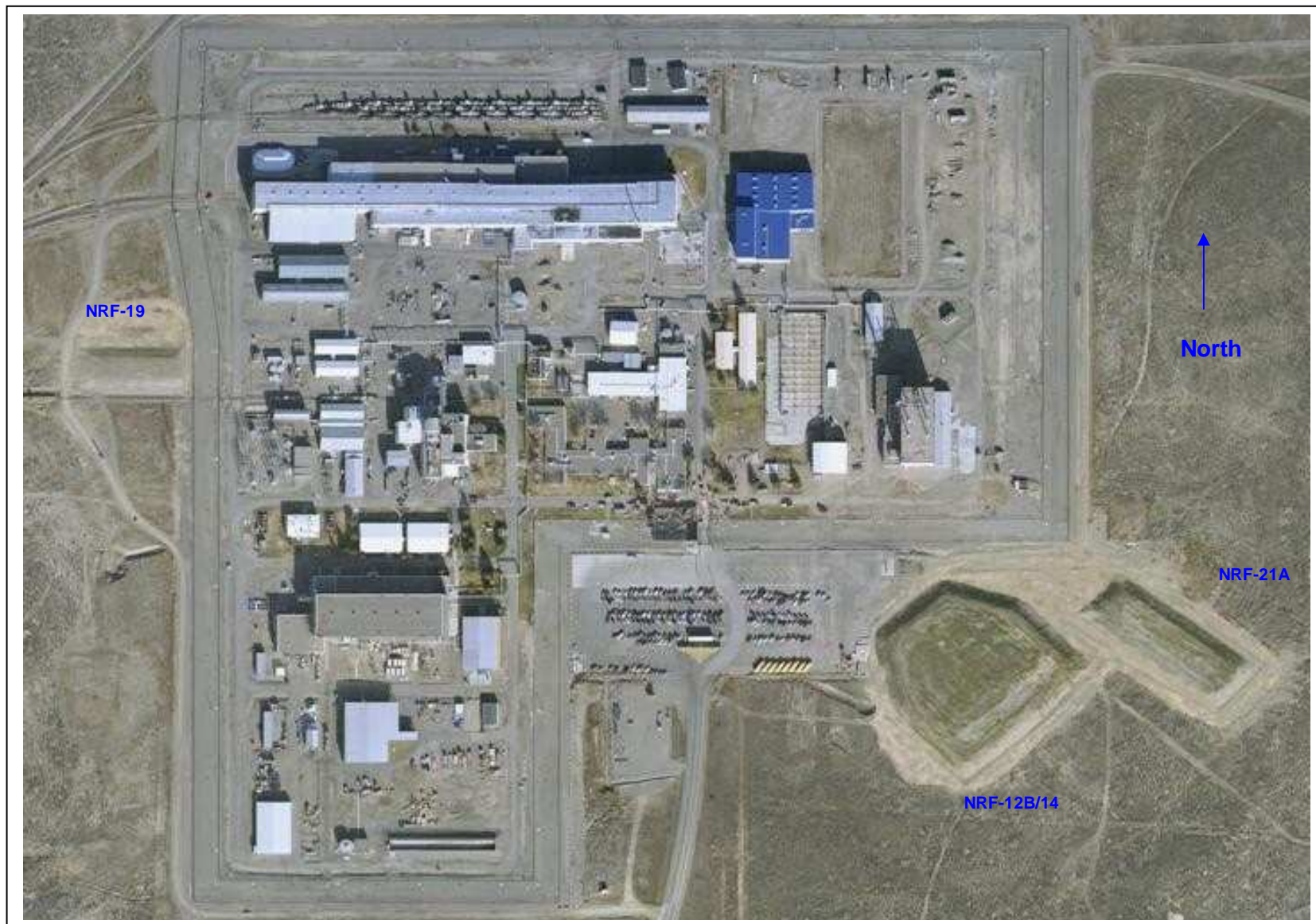
Figure 4-4 NRF-12B/14, NRF-21A, and NRF-19 OU 8-08 Engineered Cover Areas
