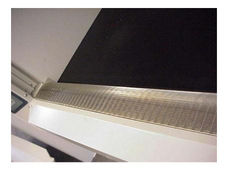
**Fig. 7** – SDSU Berkeley hood bottom supply plenum with grill.
