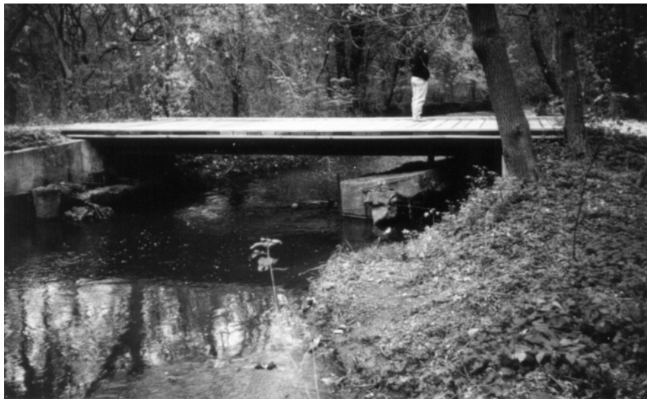
Figure 3. Spring Brook at Morris Court at Warrenville, Ill.
