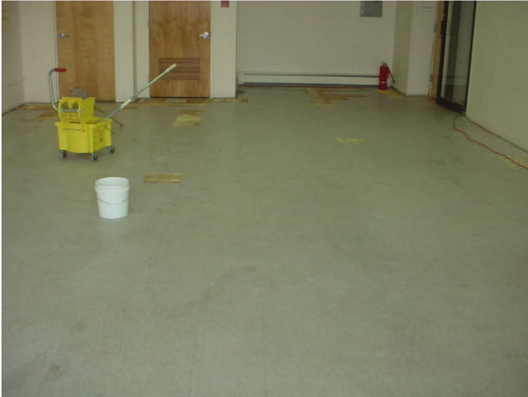
“Water Only” Washing of Floor
