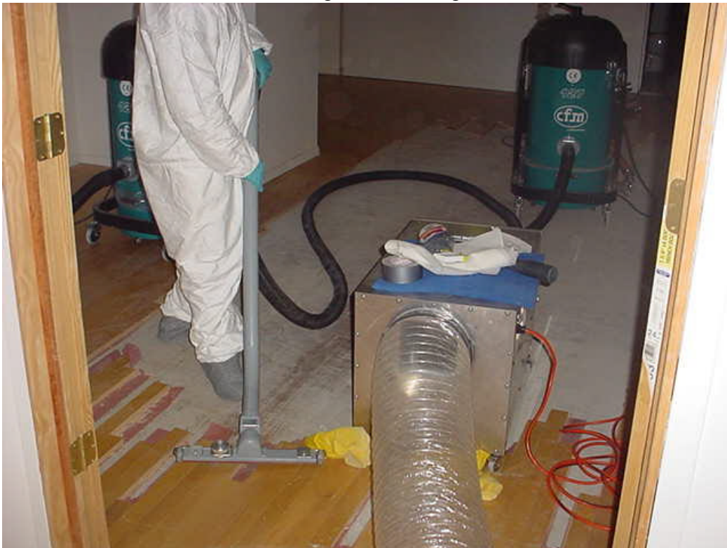
3 rd Cleaning – Vacuuming Dust
