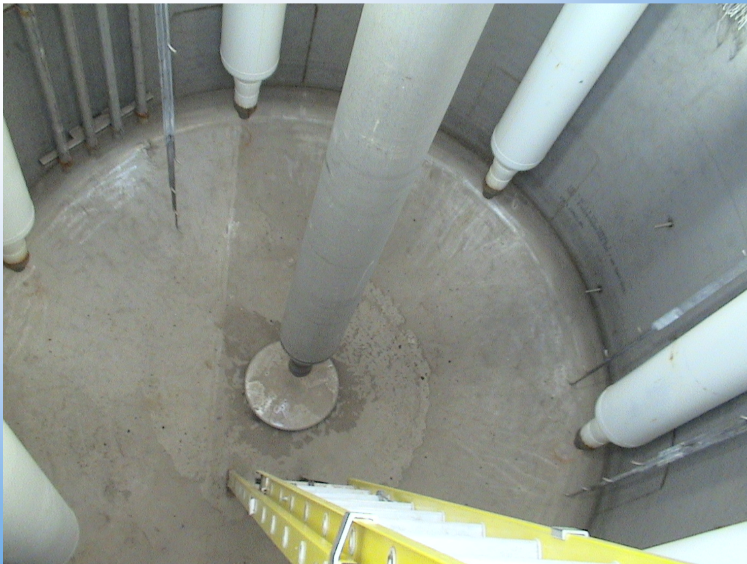
SWPF Cross Flow Filter Full Scale Test
