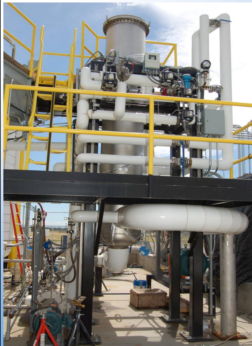
SWPF Cross Flow Filter Full Scale Test
