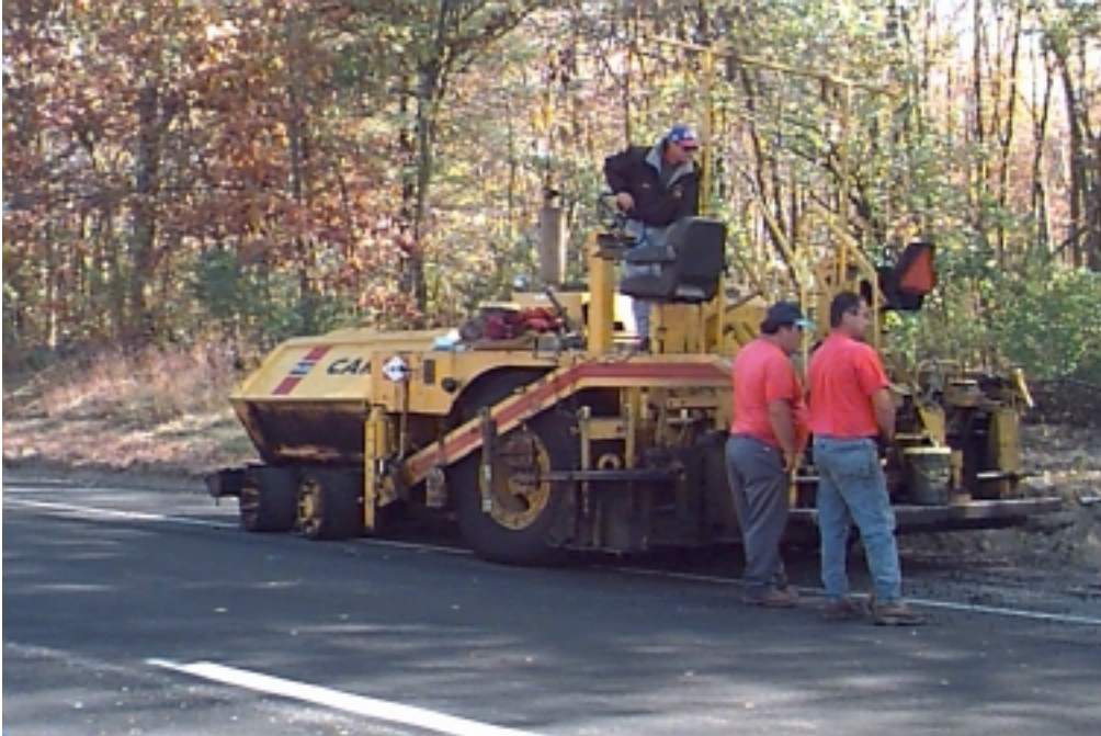
Photo #7. Blaw-Knox PF-200 Paver Used on Site 4.
