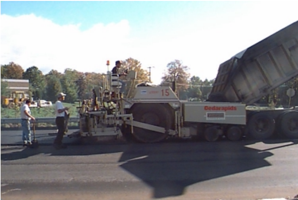
Photo #8. – Cedar Rapids CR-551 Paver Used on Site 6.
