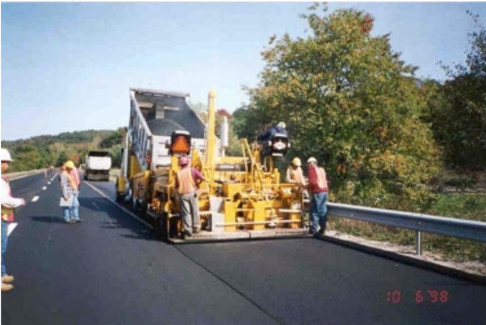
Photo #4. Blaw-Knox PF-3200 Paver Used on Site 3.
