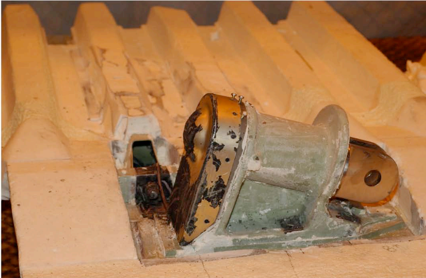
NDE mockup of bipod joint with SOFI removed.
