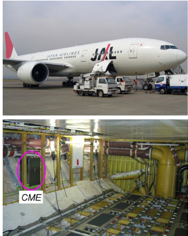
Figure 7. Forward cargo compartment of Boeing 777-200ER. Only the CME is installed on the side-wall of the forward cargo compartment.
