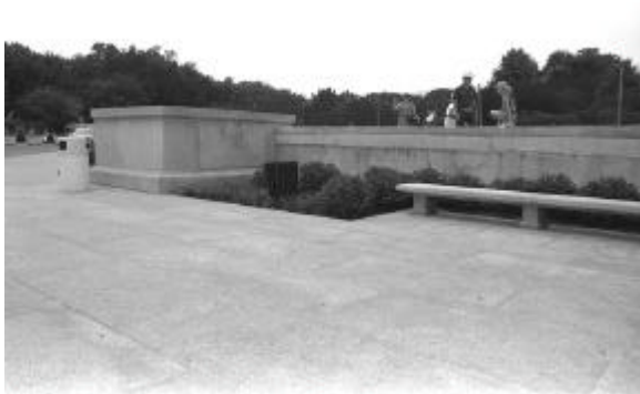
Figure 84 - Two types of trash receptacles located in the front planter by a granite bench, July 23, 1996. LINC 10-5.
