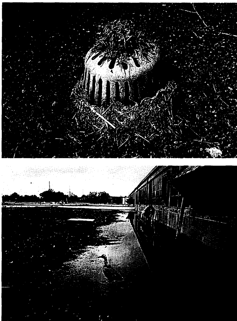
Fig. 3. Nest material can plug drain systems on roofs of buildings (top) and cause extensive flooding and damage (bottom).
