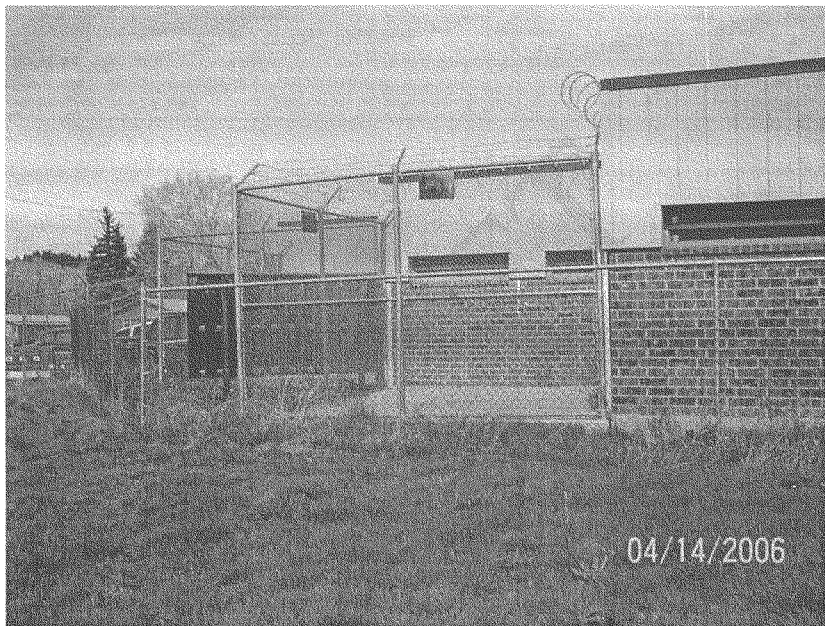
Because of the close vicinity, recreation yards may not be used for emergency evacuation as was stated at this facility
