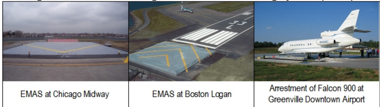
Figure 12: Illustration of Engineered Materials Arresting Systems (EMAS)
