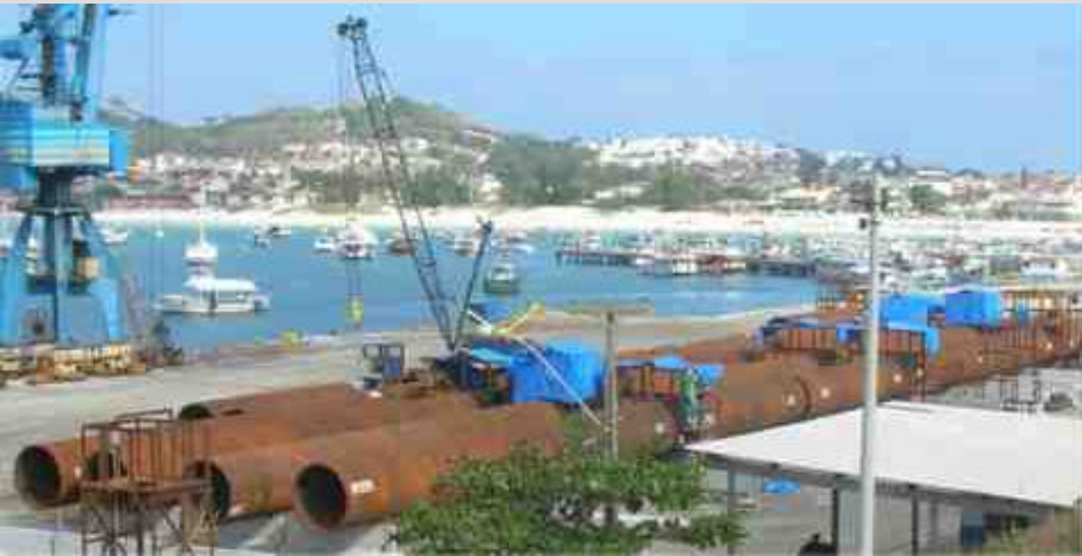
Piles – Final assembly at Porto do Forno, Cabo Frio, Brazil
