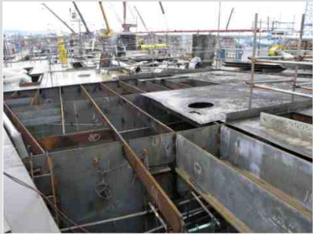
FPSO - internal work
