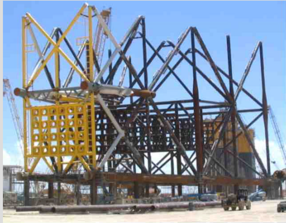
Jacket fabrication – Kiewit, Ingleside, TX
