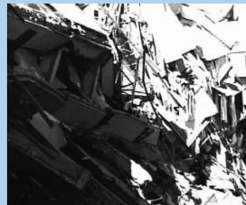
The New Orleans Riverwalk suffered extensive damage when it was struck by a bulk carrier vessel in 1996.
