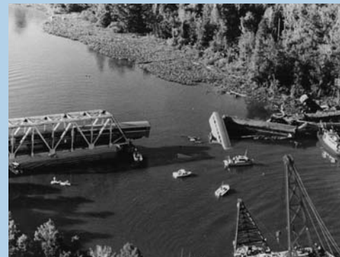
Forty-seven lives were lost when an passenger train derailed on a bridge and plunged into a bayou in 1993. Barges had previously hit the railroad bridge displacing the track.
