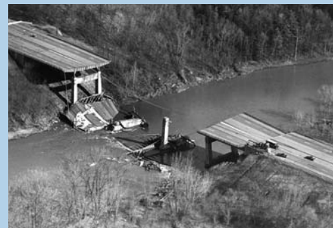
Ten people died when a New York State Thruway bridge collapsed in 1987. This was one of several NTSB-investigated accidents that resulted in improved underwater inspections of bridges and their footings.
