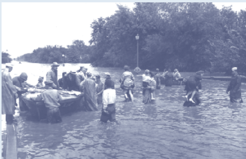
Figure 1. Women and children evacuated from ruined North Topeka were carried ashore at the north end of Topeka Avenue bridge by rescue workers (photograph courtesy of Topeka Capital Journal).
