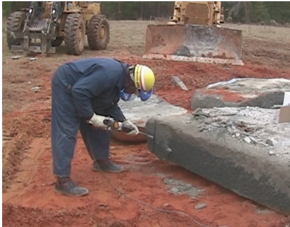
Figure 3-34. Sampling Pool 2 with electric chisel.
