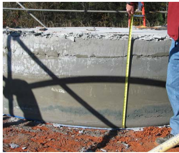
Figure 4-20. Pool 1 with form removed.
