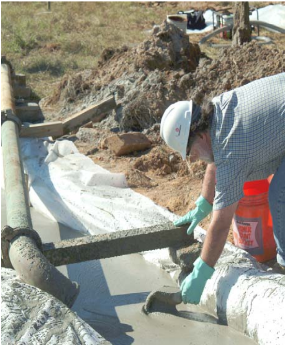
Figure 4-8. Capping grout in Trench 2 immediately after placement.
