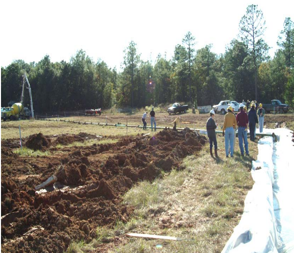
Figure 3-18. Slick line placement.
