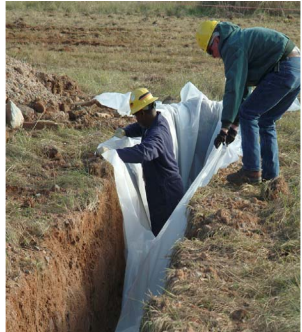
Figure 3-3. Plastic liner installation in trench.
