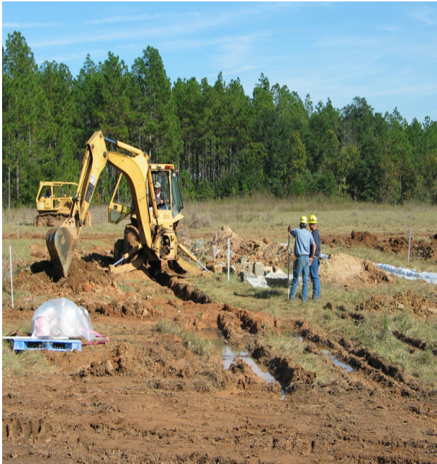
Figure 3-2. Trench form construction.
