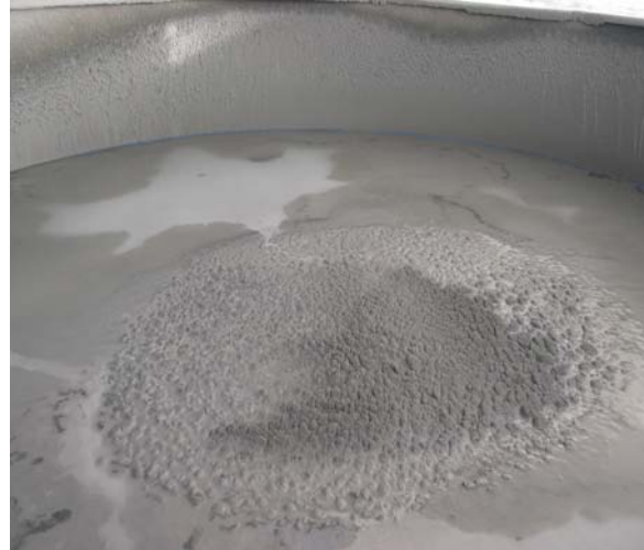
Figure 4-18. Top dressing over the second Stabilization Grout layer.
