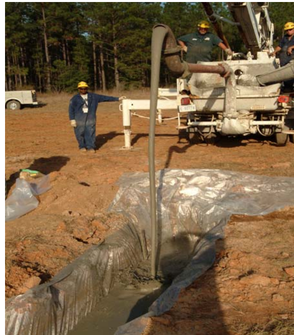
Figure 4-12. Capping grout, SRG9, discharged into Trench 3 from a ten-foot drop.
