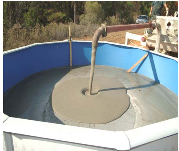
Figure 3-21. Placement into Pool 2 through a 5 inch steel pipe.
