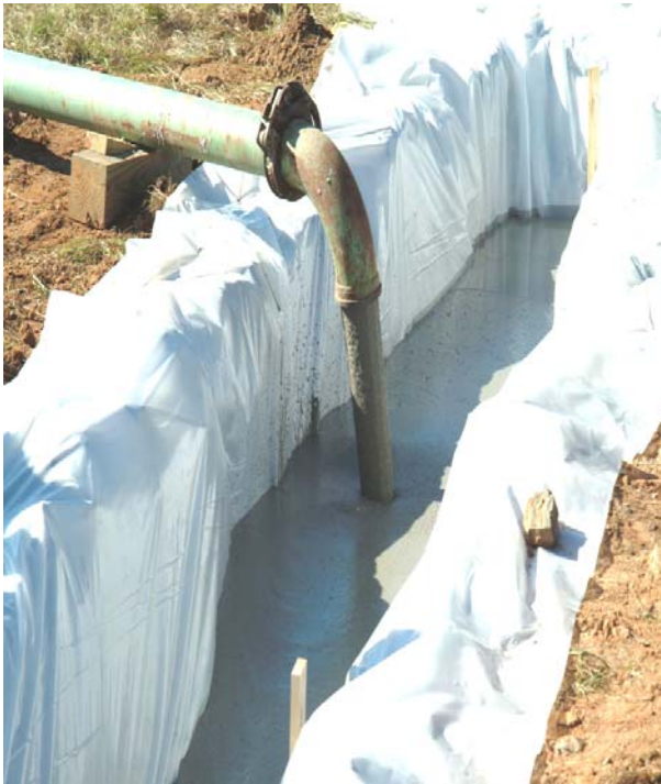
Figure 4-7. Stabilizing grout being placed in Trench 2 through a 5 inch slick line.
