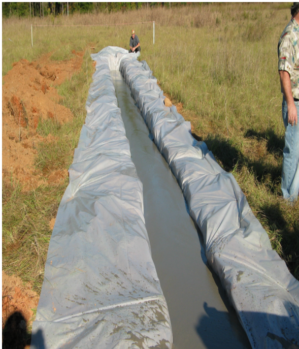
Figure 4-5. Capping grout in Trench 1 immediately after placement.
