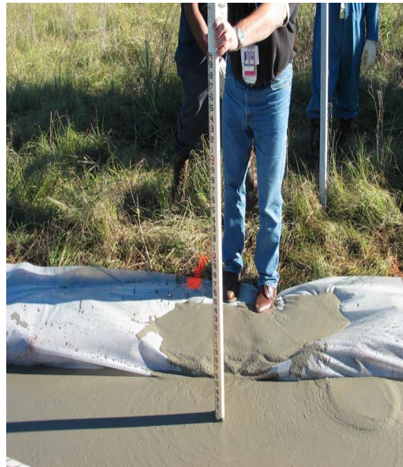
Figure 4-6. Capping grout in Trench 1 immediately after placement.
