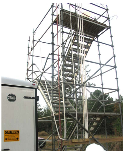
Figure 3-8. PVC pipe forms.
