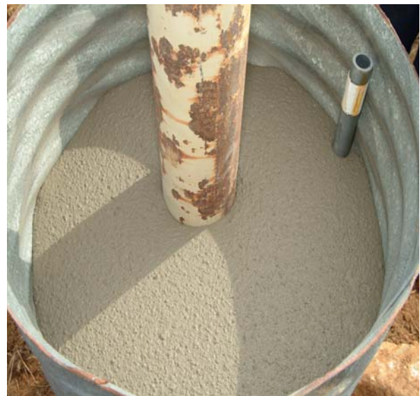
Figure 4-14. Capping grout placement in Culvert 2.
