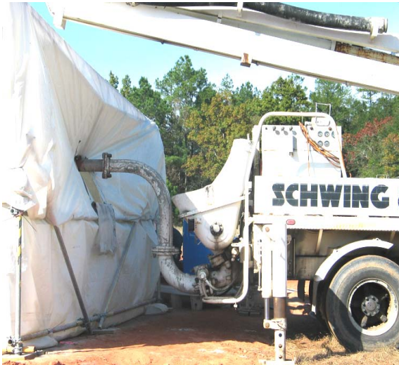
Figure 3-20. Placement into Pool 1 through a 5 inch steel pipe.
