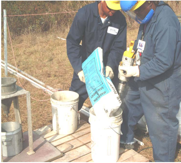
Figure 3-25. Equipment/riser grout mixing.
