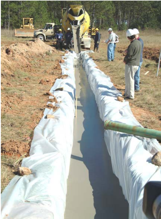
Figure 4-3. Stabilizing grout in Trench 1 immediately after placement.
