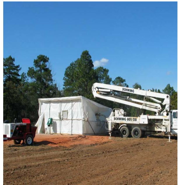
Figure 3-5. Plastic hut around Swimming Pool 1 and pump truck .
