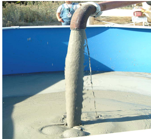
Figure 4-22. Structural grout – Pool 2.
