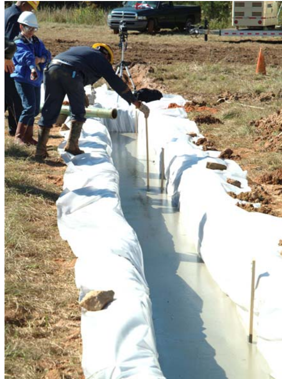
Figure 4-4. Structural grout in Trench 1 immediately after placement.
