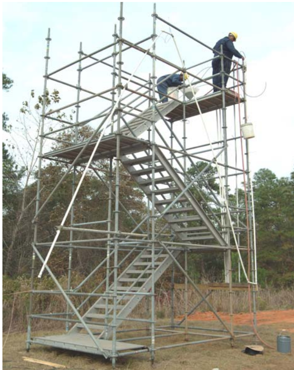
Figure 3-27. Equipment/riser grout conveyance to top of the form.
