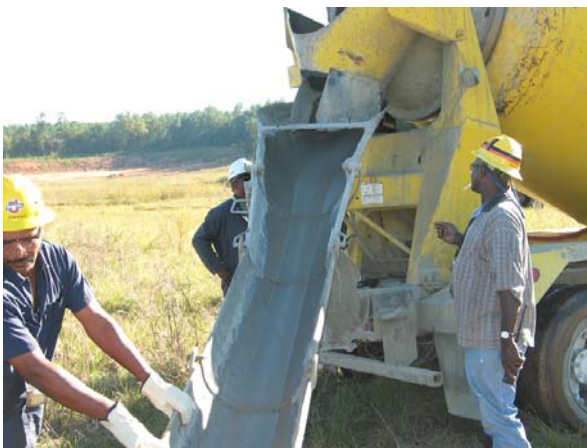
Figure 3-16. Gravity pour from a concrete truck chute into a trench form.
