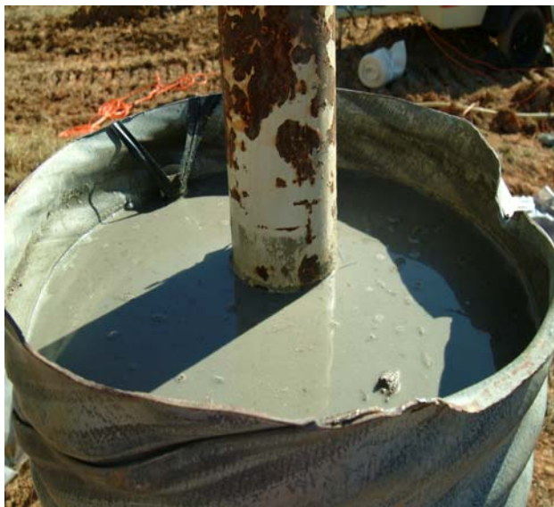
Figure 4-13. Capping grout placement in Culvert 1.
