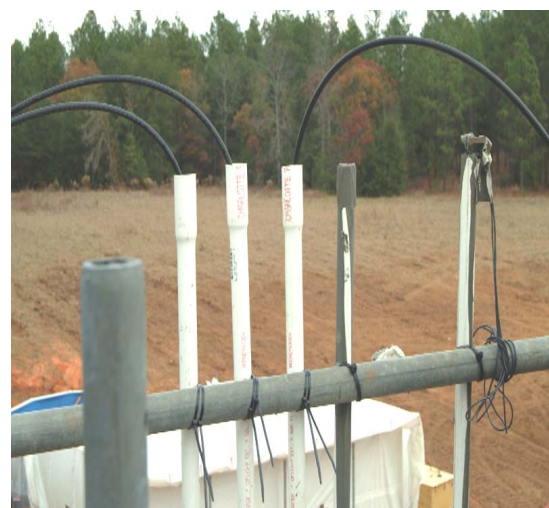
Figure 3-9. Top of one-inch PVC forms.
