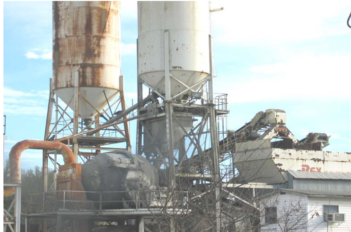
Figure 3-13. Photograph of central batch plant used to prepare grout mixes.
