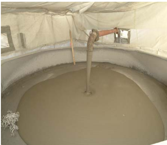
Figure 4-19. Capping grout in Pool 1.
