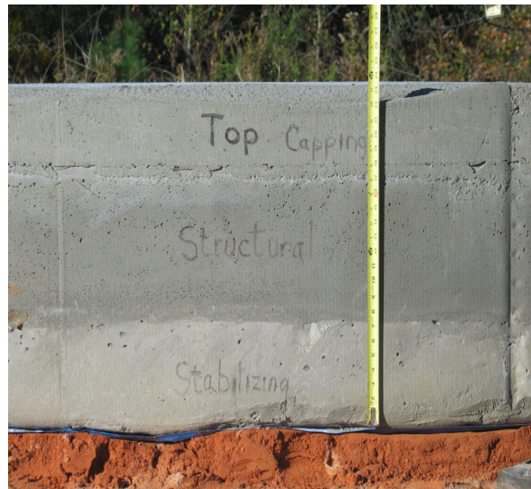
Figure 4-24. Pool 2 after the form was removed, 5 days after final pour.
