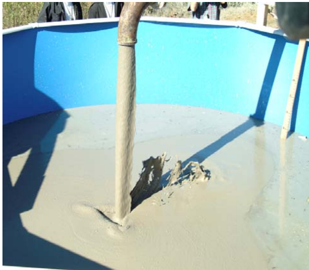
Figure 4-21. Stabilizing grout – Pool 2.
