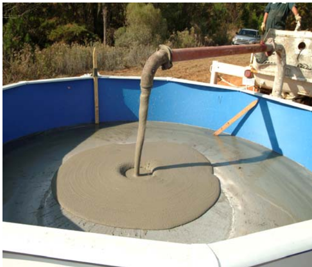
Figure 4-23. Capping grout – Pool 2.
