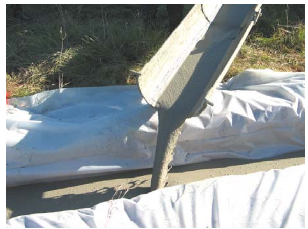
Figure 3-17. Gravity pour into a trench form from a concrete truck.
