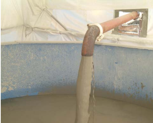
Figure 4-17. Stabilizing Grout (layer 2) placed on dry grout and C-106 simulated heel.
