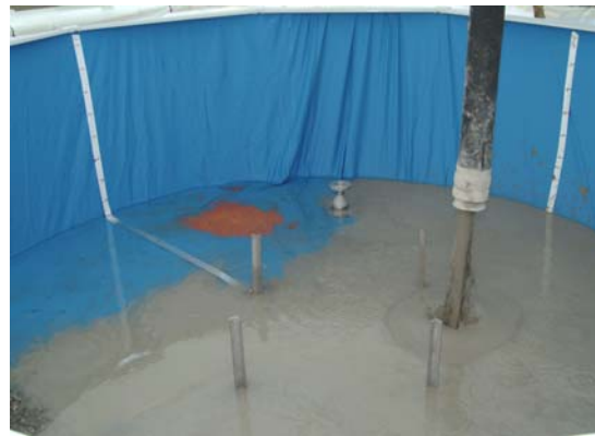
Figure 4-16. Stabilization grout as covering solid simulated heel and displacing supernate portion of the simulated heel.
