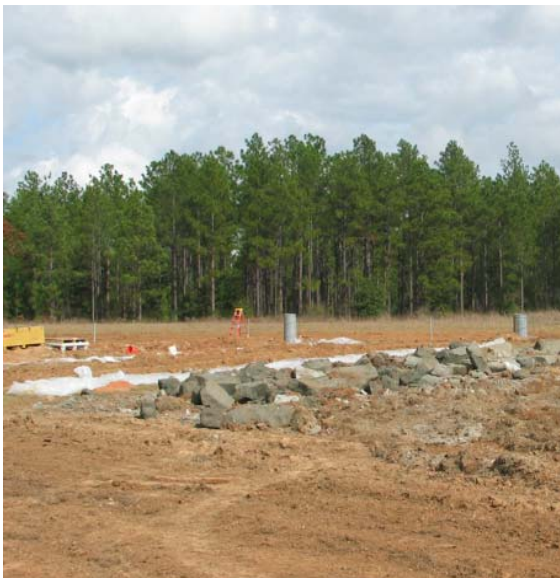
Figure 3-29. Excavation of grout placed in trench forms.
