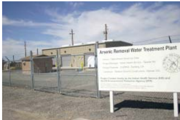
Paiute Shoshone Tribe of the Fallon Reservation arsenic removal water treatment plant
