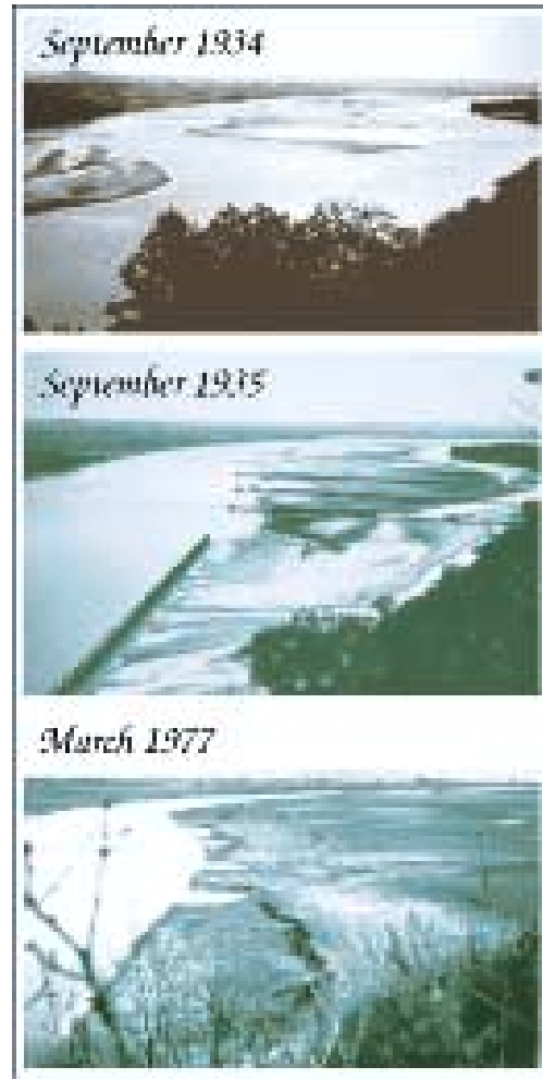
Figure 9. Channel changes. Channelization and dams have resulted in the encroachment of vegetation into the channel. These photographs collected by Norm Stuckey were taken before and after pile dikes were constructed on the Missouri River and clearly show the increase in flood plain adjacent to the channel, the decrease in width of the channel, and the change in the natural character of the channel.
