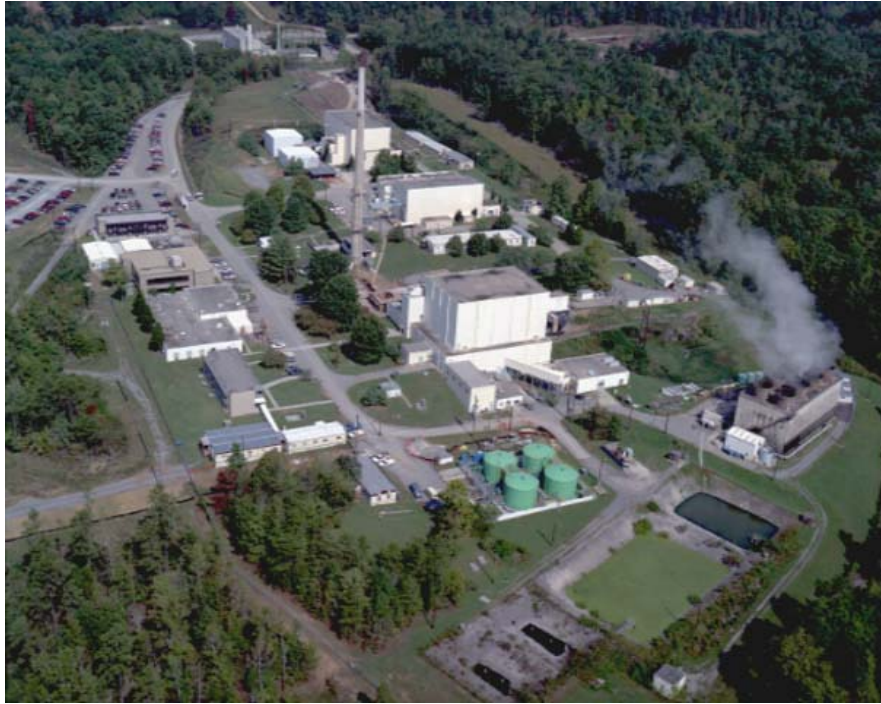
Figure 6-1. Building Complex Housing HFIR, ORNL
