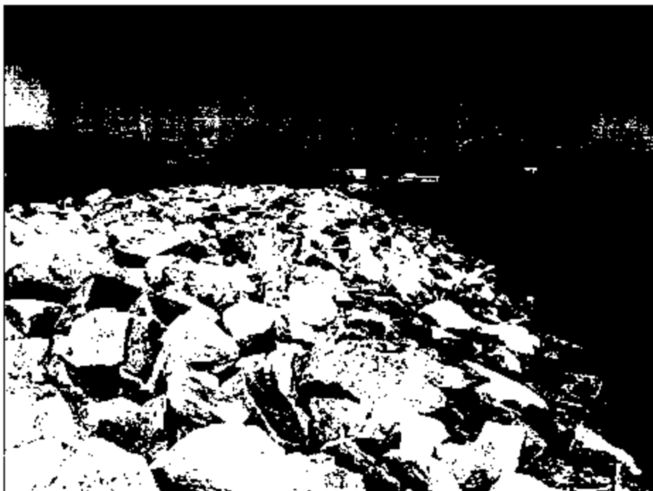
MVC - 015S: Riprap on the Potomac River shoreline at the edge of the landfill cap.
