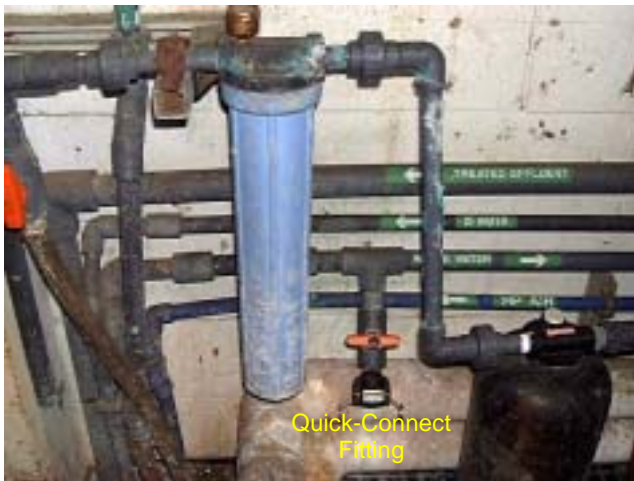
Photo No. 3 – Feeder Pipeline
