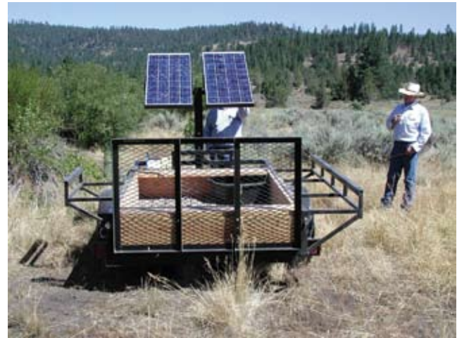
Figure 20. Mobile solar powered pump.
