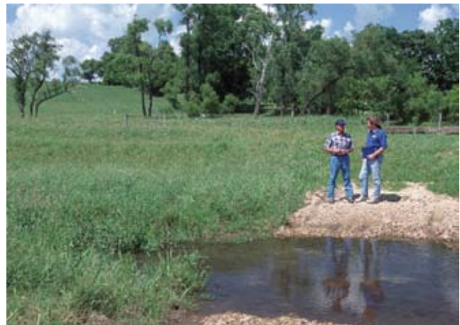
Figure 27. Hardened livestock crossing on a class 1 trout stream in Columbia County, Wisconsin (2000). (Photo by B. Nichols, NRCS.)
