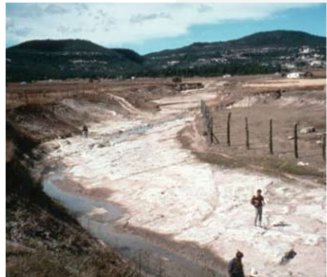
Figure 2. Bank erosion caused by a bedrock channel bottom. (Photo by J. Staats, NRST.)
