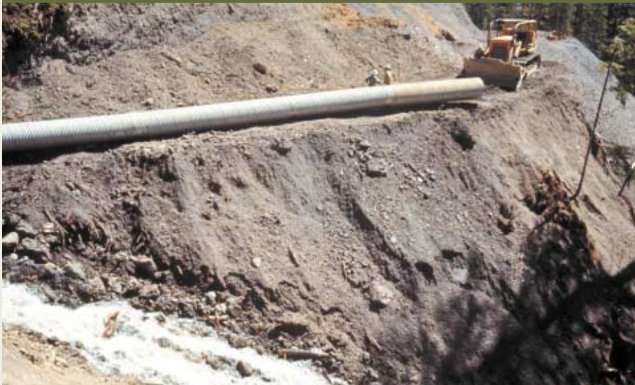
Figure 44. Forest road construction in the 1970s in Olympic National Forest.
