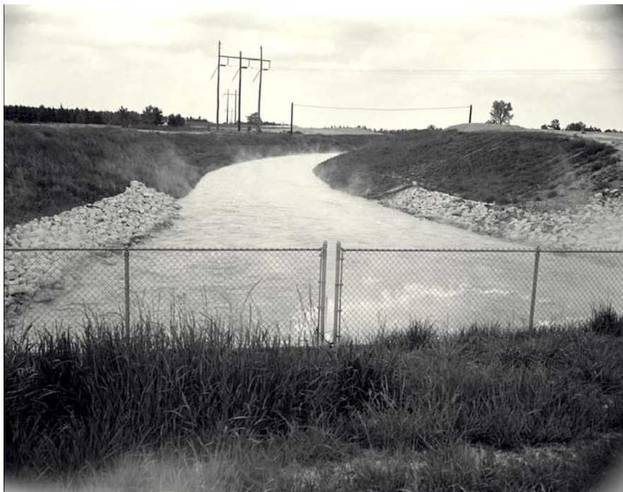
Figure 9 Effluent Canal, P-Area Looking downstream toward Par Pond (DPSPF-7459-2) 5/5/1961
