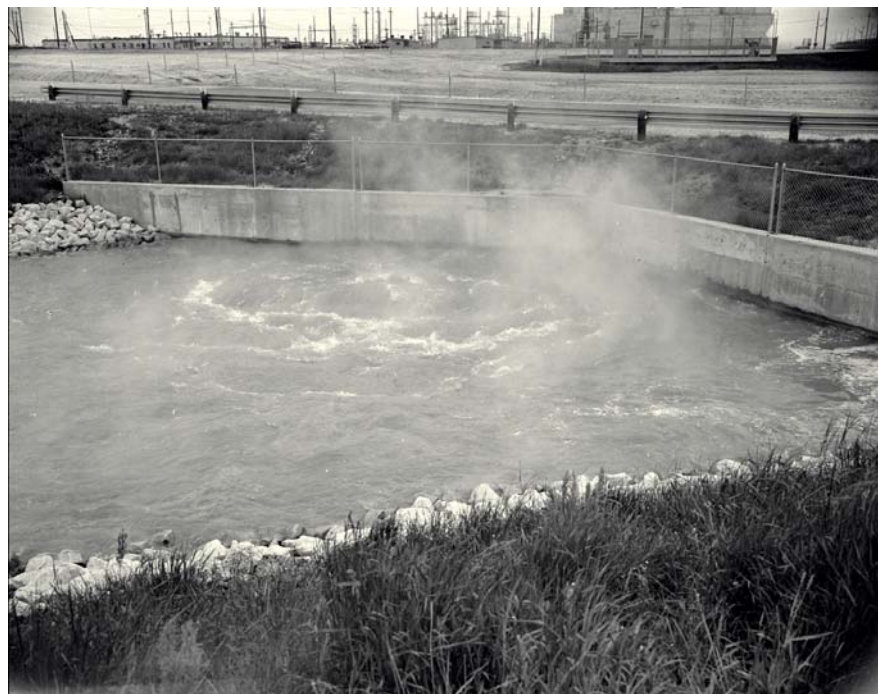
Figure 7 Effluent Canal, P-Area Discharge Point to Par Pond Completed (DPSPF-7459-1) 5/5/1961
