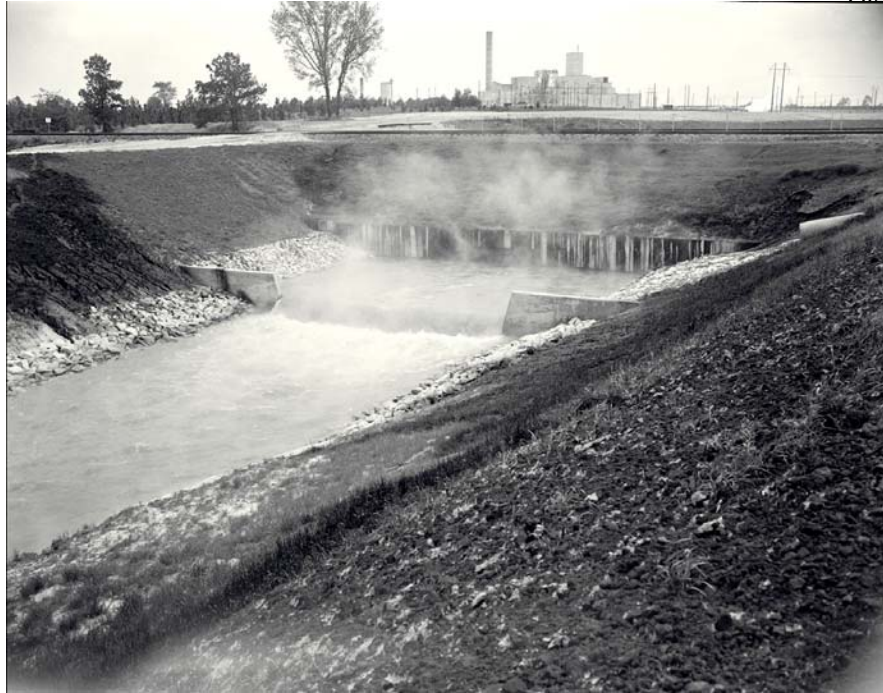
Figure 8 Effluent Canal, P Area Completion of P Area Canal to Par Pond (further downstream from P Area, heading toward Par Pond) (DPSPF-7459-5) 5/5/1961
