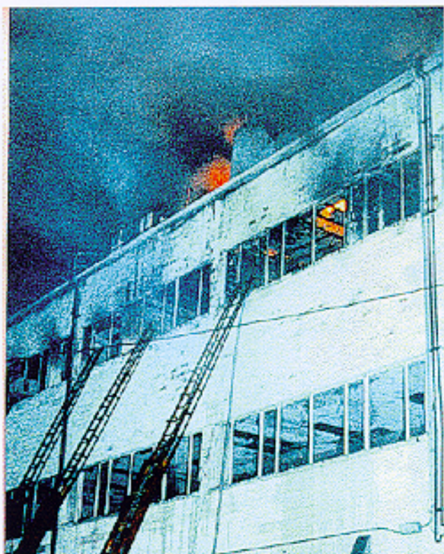
3-3 (top) and 3-4 (bottom): Commercial office building fire, Ventura Blvd., Sherman Oaks
