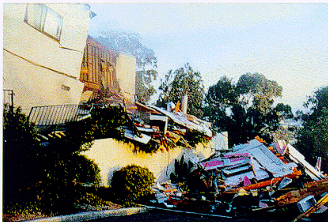
3-13: Total collapse of end units of condominium, Granada Hills.
