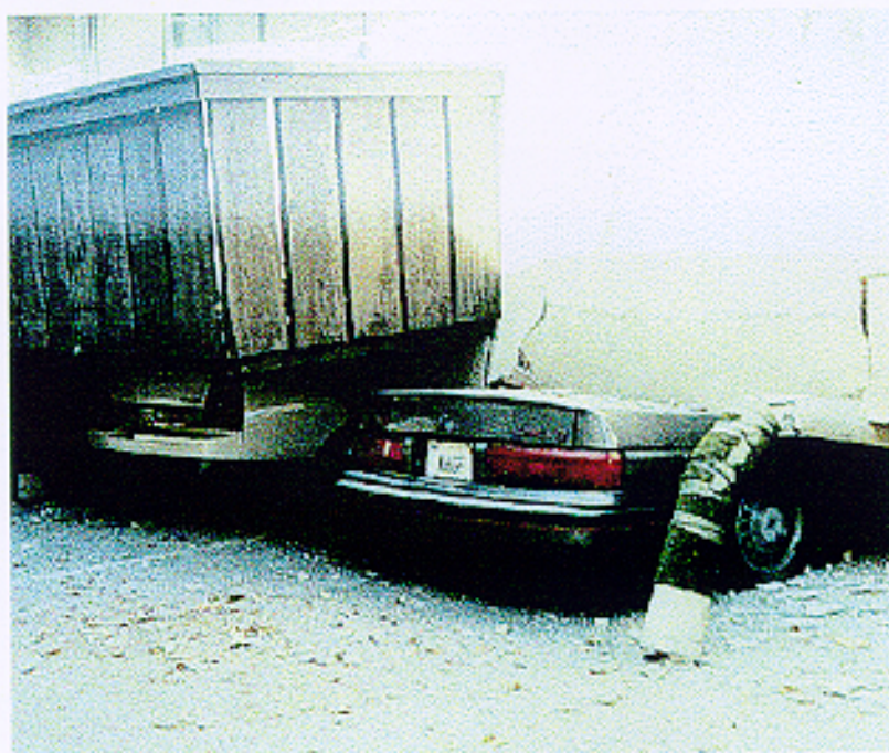
3-19 (top) and 3-20 (bottom): Northridge Meadows Apts. collapse of structure from soft first story parking garage. Three story building, 16 killed, hundreds rescued, 9565 Reseda Blvd.
