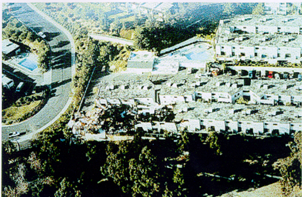
3-12: Aerial view, collapsed condominium, Granada Hills.
