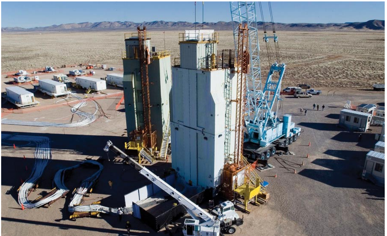
Towers at the Nevada Test Site, where the test rack for a subcritical test was assembled before being placed downhole
