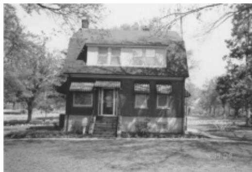
The lodge was constructed in 1934. The first story is brick and the dormered second story is frame and stucco, with a concrete foundation and an asphalt shingle gambrel roof. The second story has stucco gables with exposed wood loosely imitating half-timber English tudor. The lodge contains six rooms, an office, a basement, and a front porch which was enclosed in 1952. No director has resided in the lodge since January 1991, and the building is now used as an administrative office.
