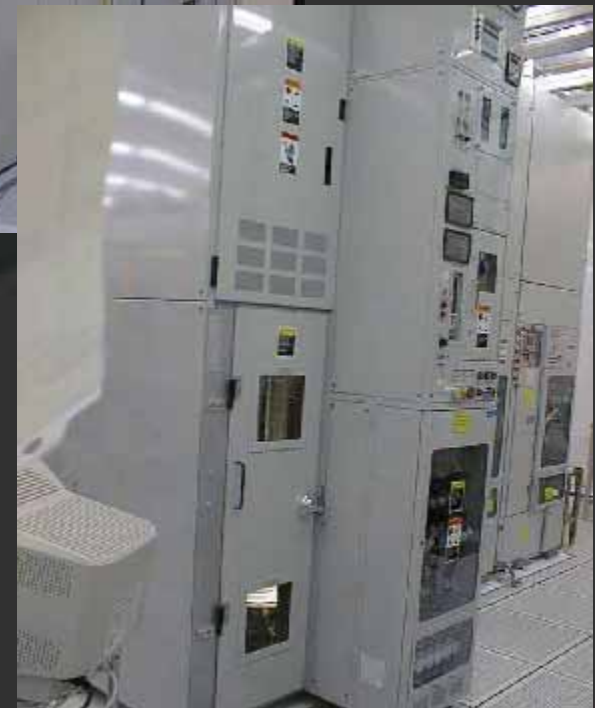
Vertical Furnace - 628 to 474 scfm
