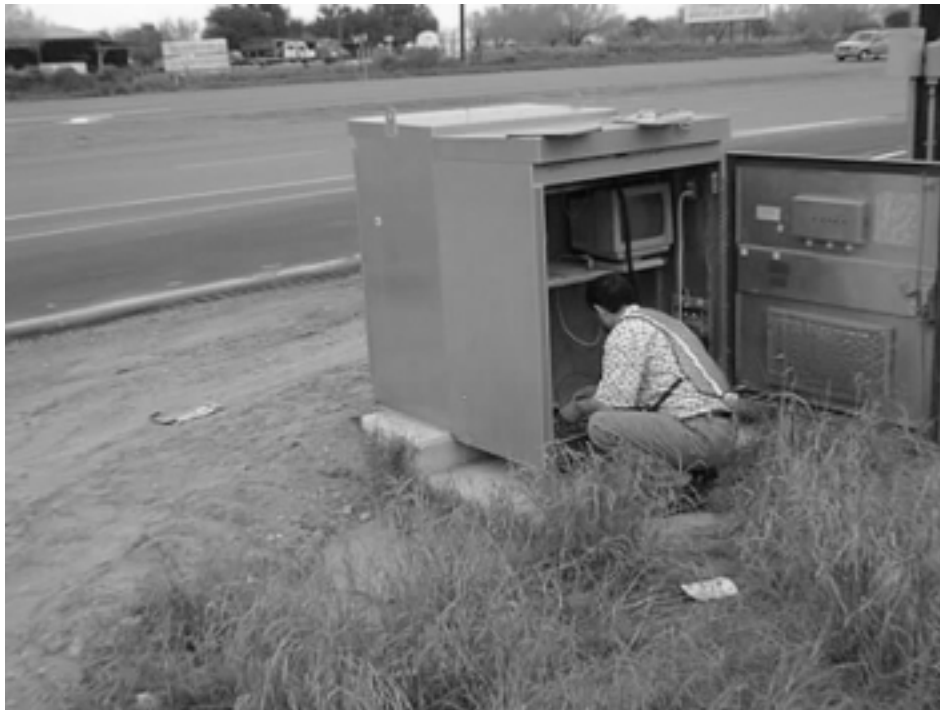
Figure 2. Cabinets Located Back to Back at the Intersection
