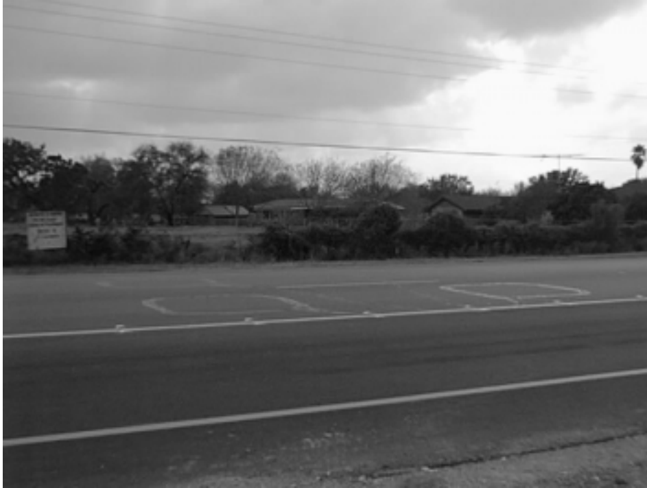
Figure 1. Loops Placed on the Eastbound Approach
