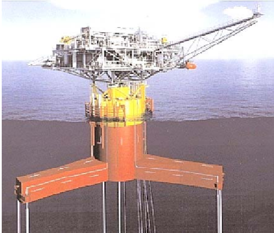
Figure 26 – Typhoon TLP (Payload 5,000 tonnes, Water Depth 2,100ft) 74
