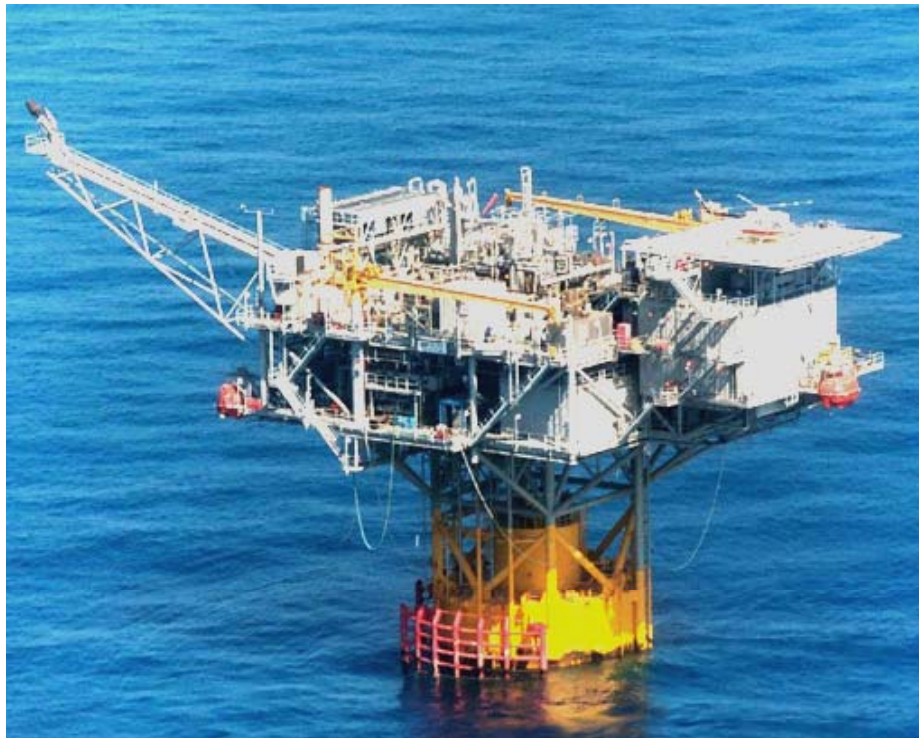
Figure 23 – Allegheny TLP (Payload 4,000 tonnes, Water Depth 3,300ft) 73
