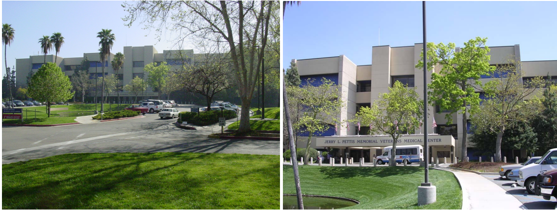
Figure 17. Wide-angle (left) and close-up (right) exterior views of 11201 Benton St. (photos by Janise Rodgers and François Dunand)
