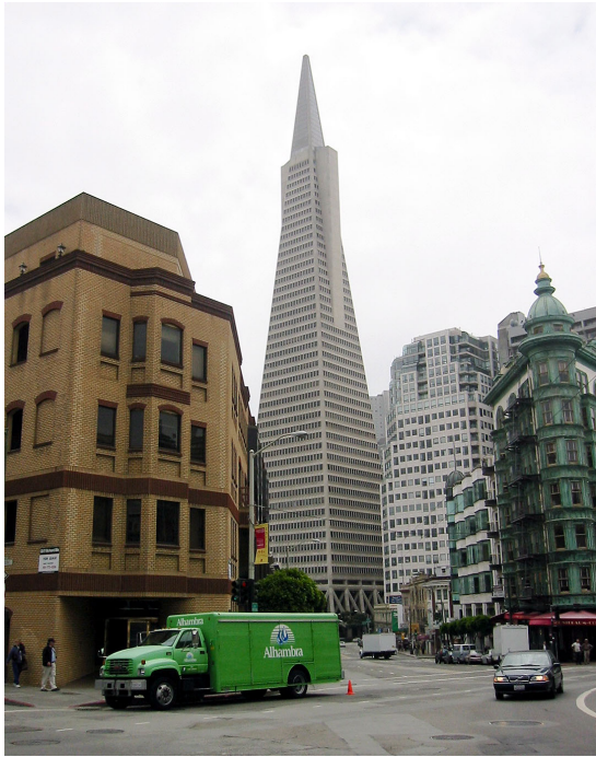
Figure 11. Exterior view of 600 Montgomery St. (photo by Dan Radulescu)
