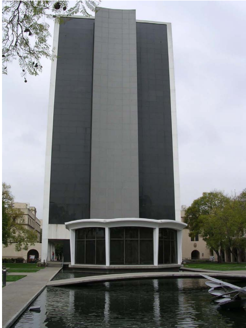
Figure 24. Exterior view of Millikan Library (photo by François Dunand)
