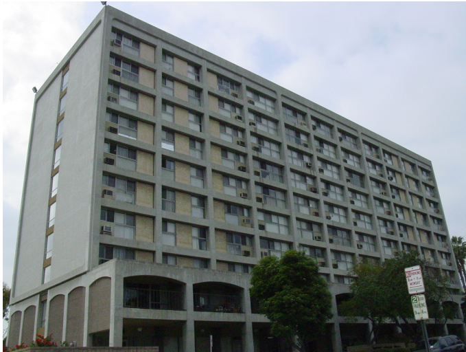
Figure 3. Exterior view of 7215 Bright. Ave. (photo by Janise Rodgers)
