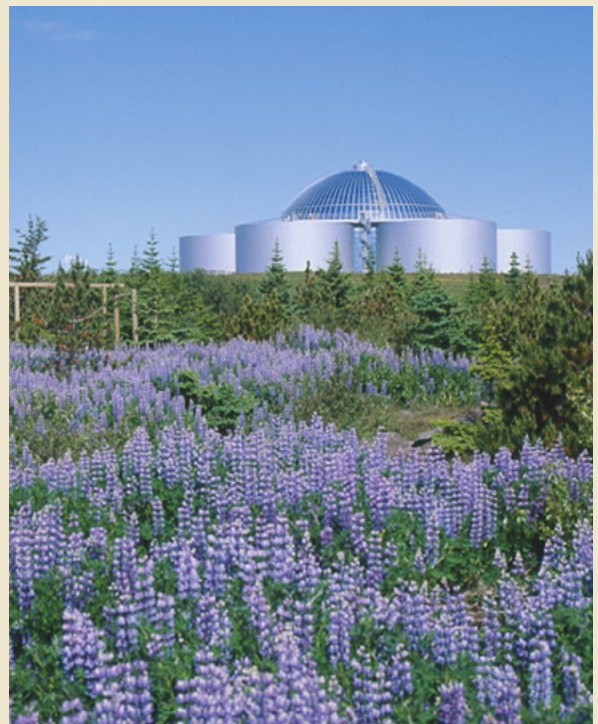
Exterior of rotating restaurant on top of hot-water storage tanks in Reykjavík, Iceland. (Photograph by Gudmundur E. Sigvaldason, Nordic Volcanological Institute, Reykjavík, Iceland.)
