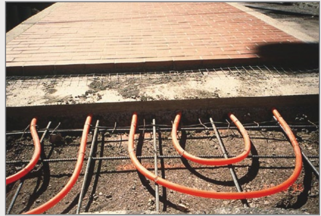
Tubing carries geothermal water whose heat melts snow on this walkway in Klamath Falls, Oregon. (Photograph by Kevin Rafferty, Geo-Heat Center, Oregon Institute of Technology.)
