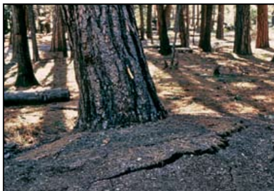
Figure 23 New lean soil cracking
