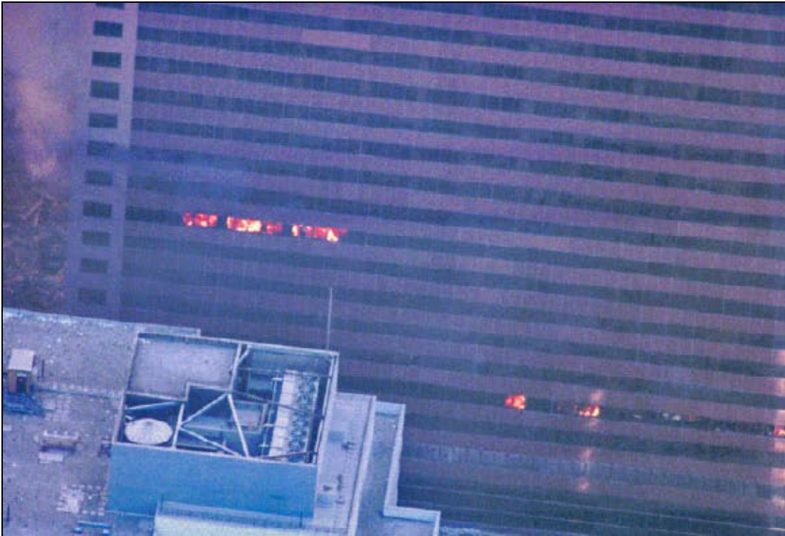
Photo 22. The north side of Building 7. Fires are on the 7th and 12th floors. (Courtesy of NIST.)
