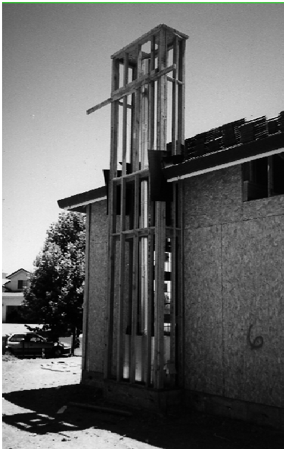
Figure 7-7 Factory-built flue and light-frame enclosure.
