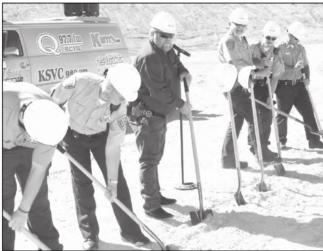
Sheriff's Department deputies joined other dignitaries in groundbreaking for new Sanpete County Jail last Friday.
