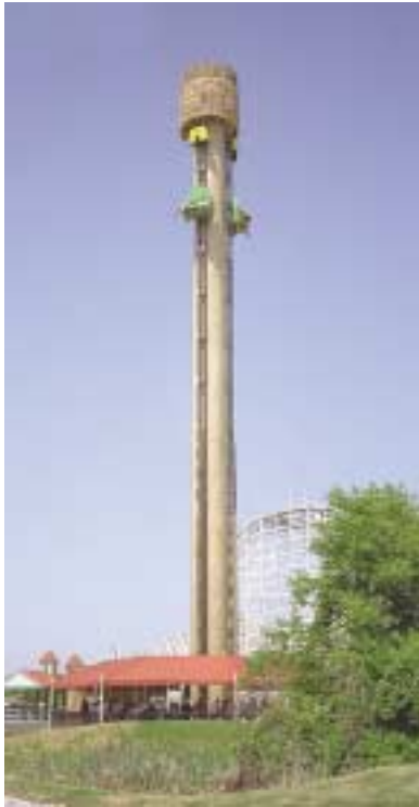
The Tower of Doom is located at Six Flags of America, Largo, Maryland. The riders plunge into free fall from a height of 150 feet. This ride has magnetic brakes to cushion the descent.
