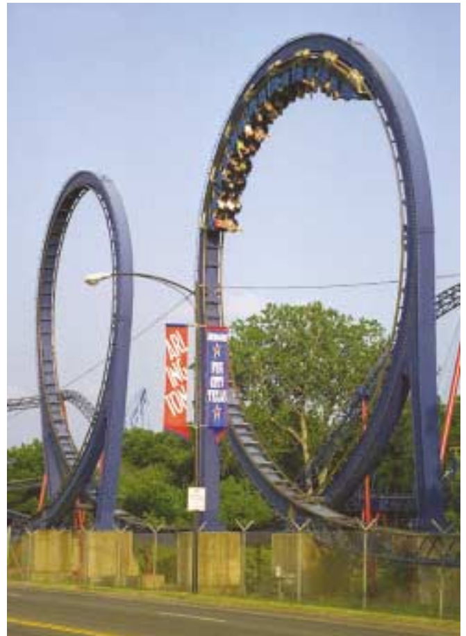
The Shock Wave, built in 1978, was the first coaster to feature two consecutive vertical loops. It still runs without shoulder restraints. It is located at Six Flags Over Texas, Arlington, Texas.
