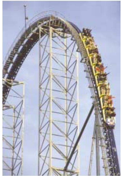
Cedar Point's Magnum XL-200 has a lift hill that is over 200 feet tall. The coaster has no loops in its out-and-back course. The Magnum XL-200 is located at Cedar Point, Sandusky, Ohio.
