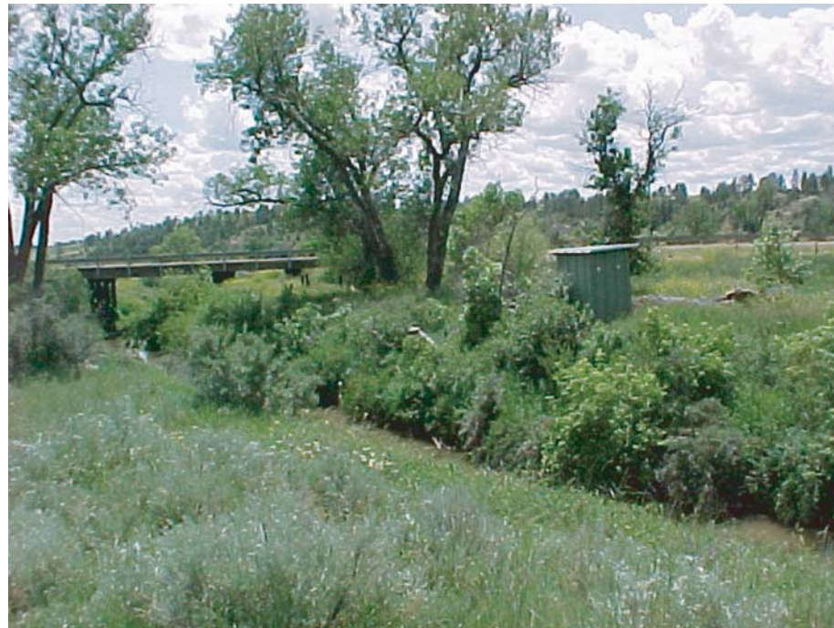
Figure H5. Otter Creek at Ashland site from right bank at cross section 2 looking upstream at gaging station and bridge. Date of photograph unknown.
