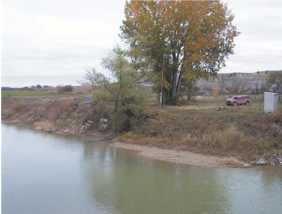
Figure D7. Tongue River below Brandenburg Bridge site from bridge looking downstream at right bank, gaging station, and irrigation diversion. Photograph taken October 23, 2002.
