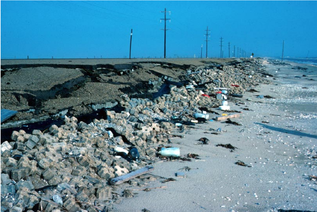
Figure 24. Storm waves in the Gulf of Mexico destroyed the interlocking block revetment constructed to protect Louisiana State Highway 82 near Peveto Beach (Fig. 3). The revetment structure was replaced with 85 segmented breakwaters between Constance Beach and Holly Beach (Fig. 3).
