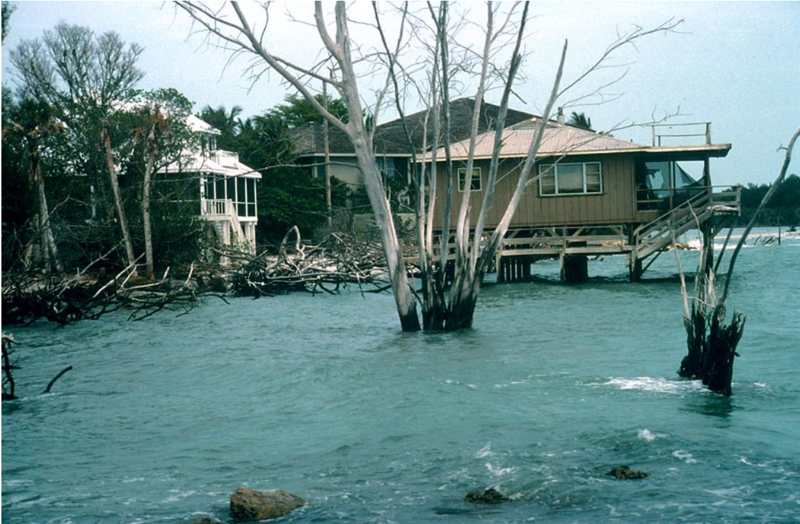
Figure 14. Erosion of the Gulf shore eventually destroyed this beach house at Captiva Island, Florida.
