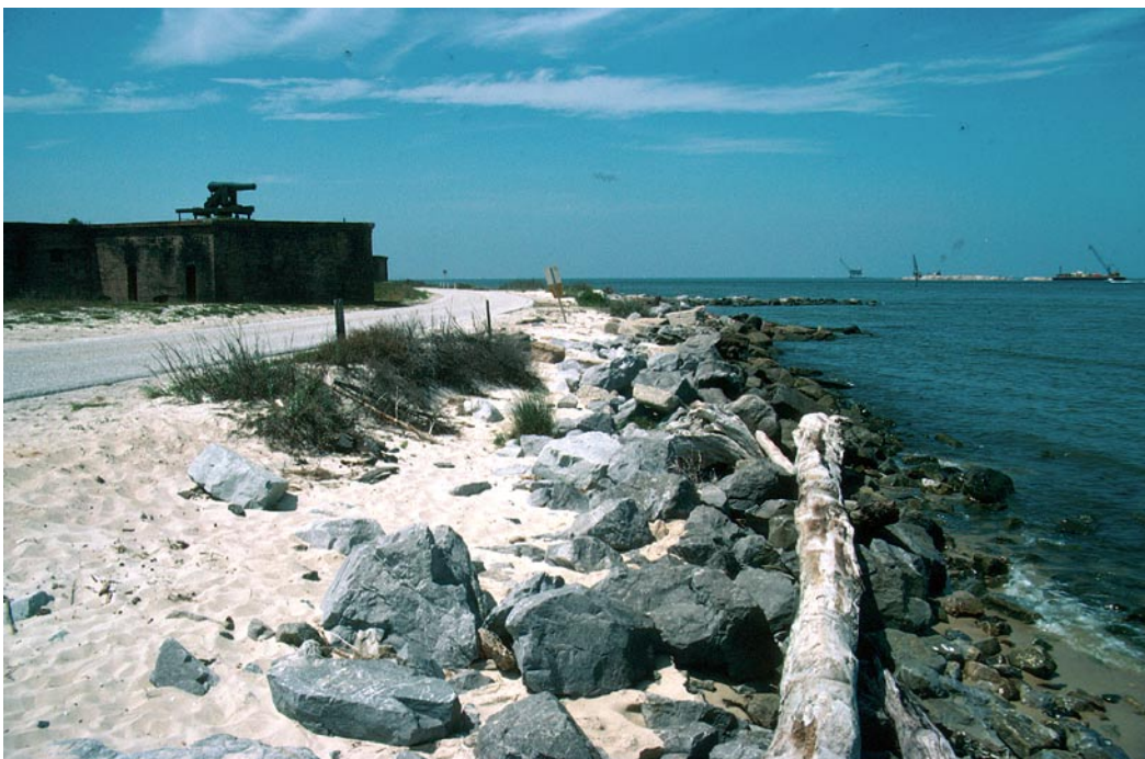
Figure 23. Rock revetments and groins have been used to control beach erosion at Fort Gaines on the east end of Dauphin Island, Alabama.
