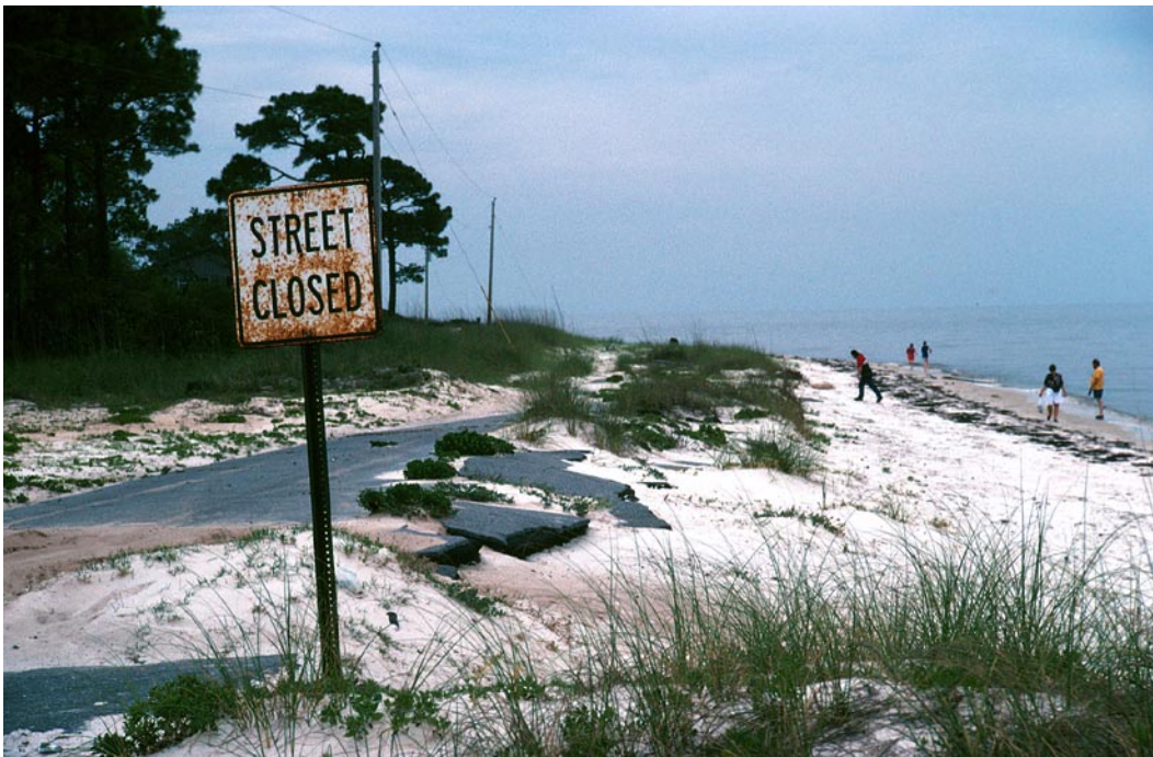
Figure 15. Even where wave energy is normally low, episodic erosion during storms is capable of destroying roads and eliminating the beach. This example of erosion along the low energy coast is from Lighthouse Point, Florida.
