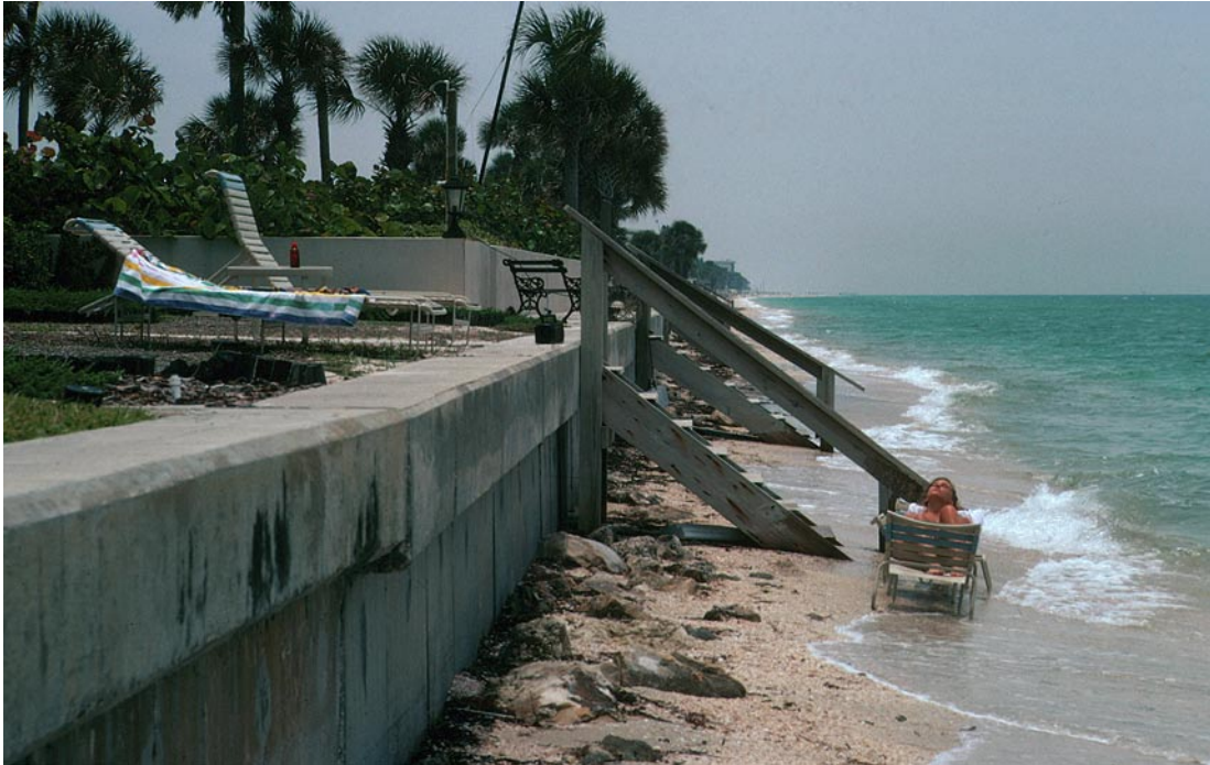
Figure 16. This narrow eroding beach in front of a seawall near Clearwater, Florida was used for recreation before beach nourishment.
