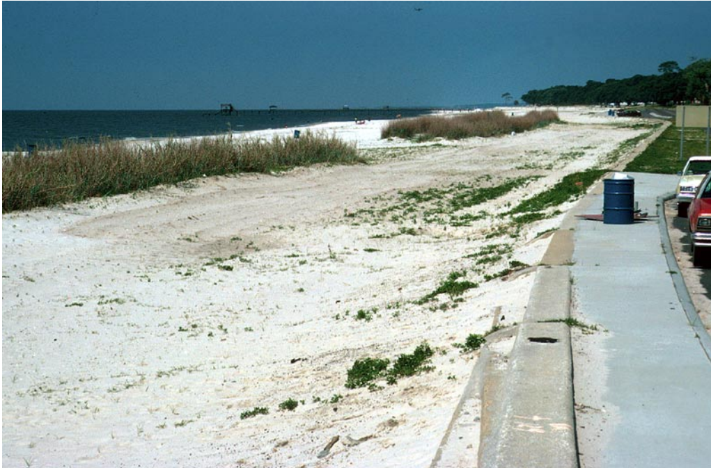
Figure 19. The seawall along U.S. 90 at Biloxi, Mississippi extends for nearly 27 miles. This reinforced concrete structure provides protection from minor storms and high water but it was unable to prevent massive destruction and death caused by Hurricane Camille in 1969.
