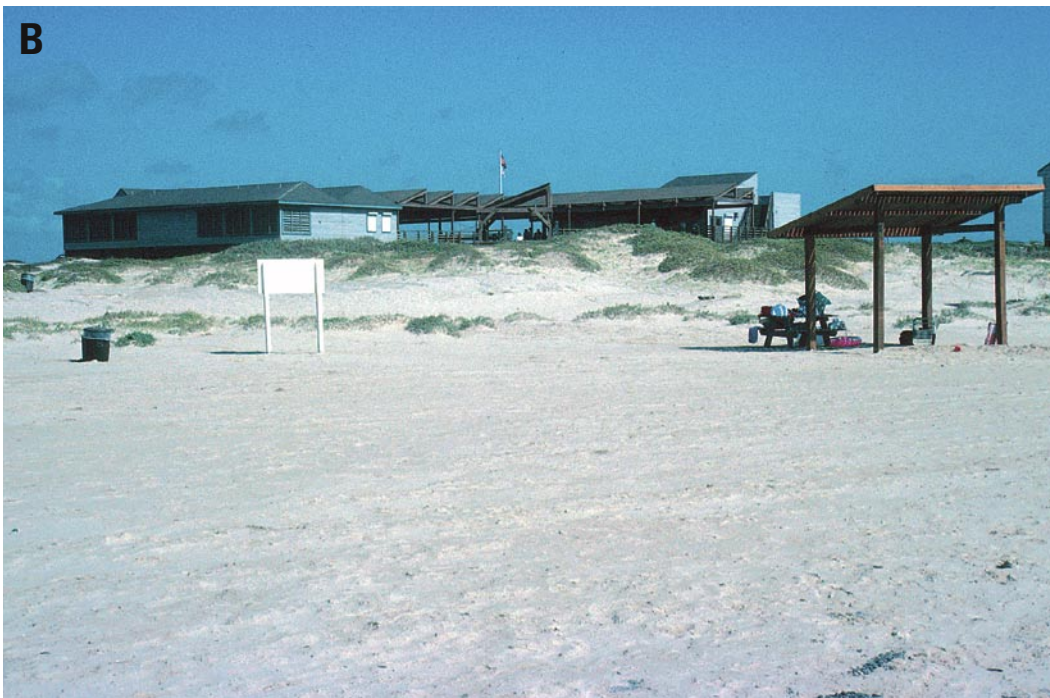
Figure 26. Visitor's center at Padre Island National Seashore, Texas in 1982 and 1992. The concrete reinforced structure built on the beach was torn down and a wooden structure was built landward of the dunes.
