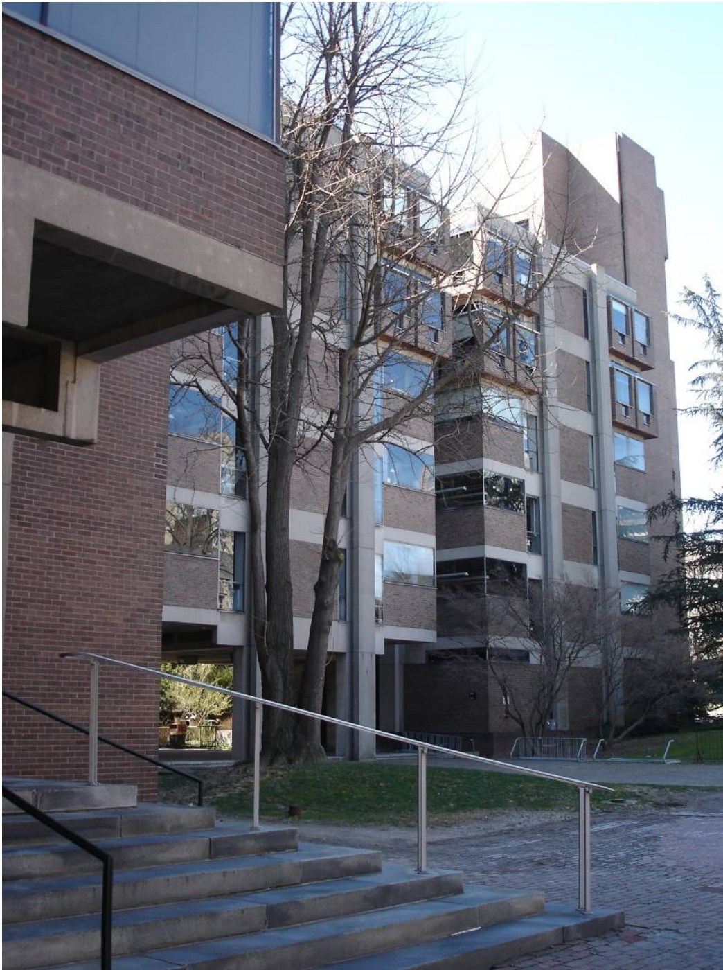
Richards (foreground) and Goddard (rear) buildings, looking southwest John Dixon Hunt, photographer, March 2008
