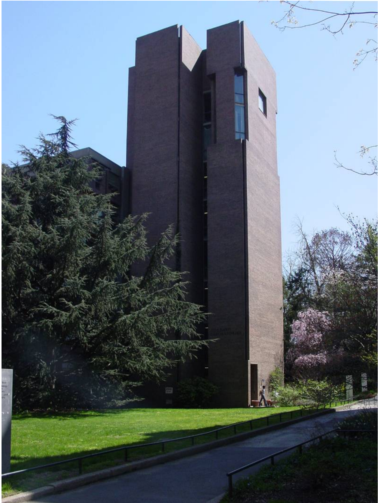
Western tower, Goddard Building, looking southeast from Hamilton Walk Emily T. Cooperman, photographer, April 2008
