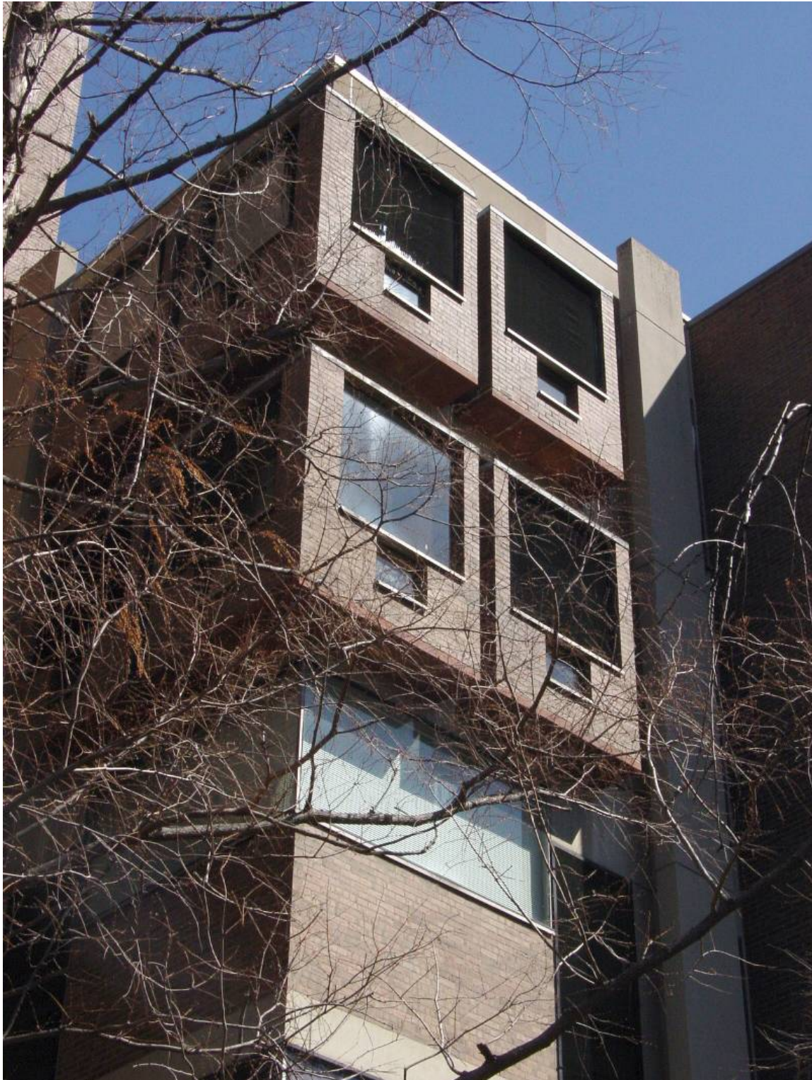
Upper floors of Goddard Building, eastern laboratory and classroom tower, looking east, showing projecting carrel volumes Emily T. Cooperman, photographer, March 2008
