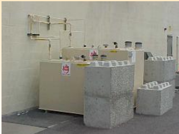
#1 - Bulk tanks ready to dispense needed material
