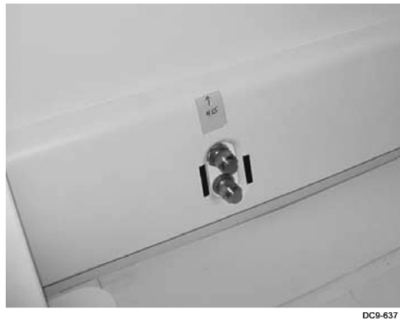
Figure 14. Multi-User Overboard Vent
