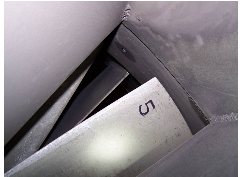
Probe Installation -Fan Interior
